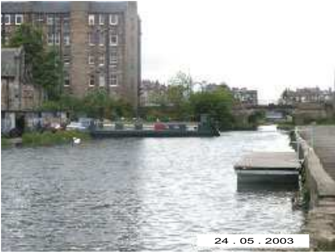
Plate 1. (above) Leamington Wharf looking east. The lower courses of the north wall are the original 1818 revetment. The original width of the canal is represented by the edge of the track, centre left, and the north wall.
