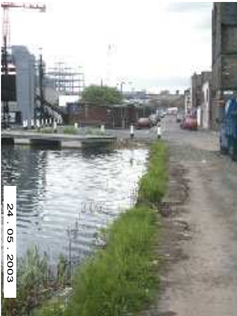
Plate 3. (below) Masonry of the original 1818 masonry revetment wall adjacent to the re-located lift bridge. Immediately in front of the modern pontoon is the location of the sunken barge that is shown on the 1853 Ordnance map.
