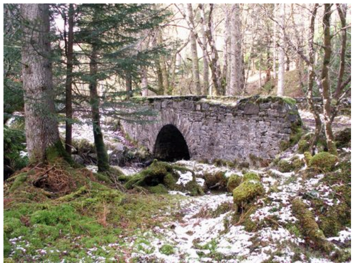
The southern late 19 th century bridge, deep in the woods. Feature 1.
