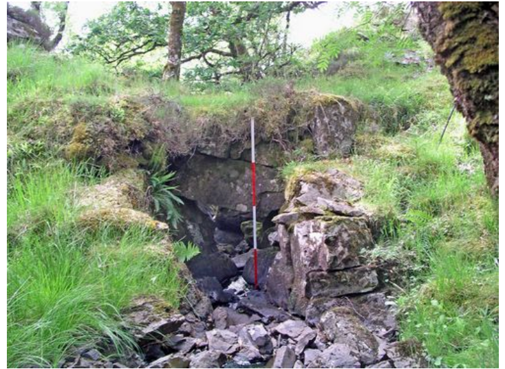
Donald Dubh's Bridge, crossing the same tributary of the Mingarry burn at the western edge of Mingarry, viewed from north. Feature 84.
