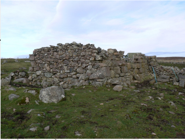
View of S wall showing altered construction
