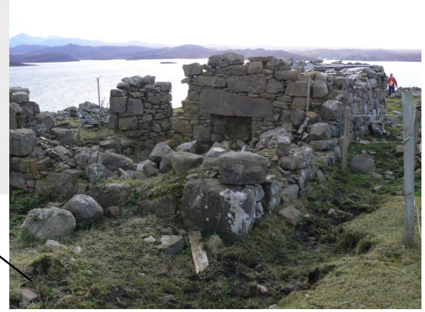
View from NW looking across ruin and showing fireplace with large lintel stone
