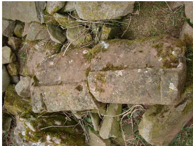
Moulded sandstone blocks
