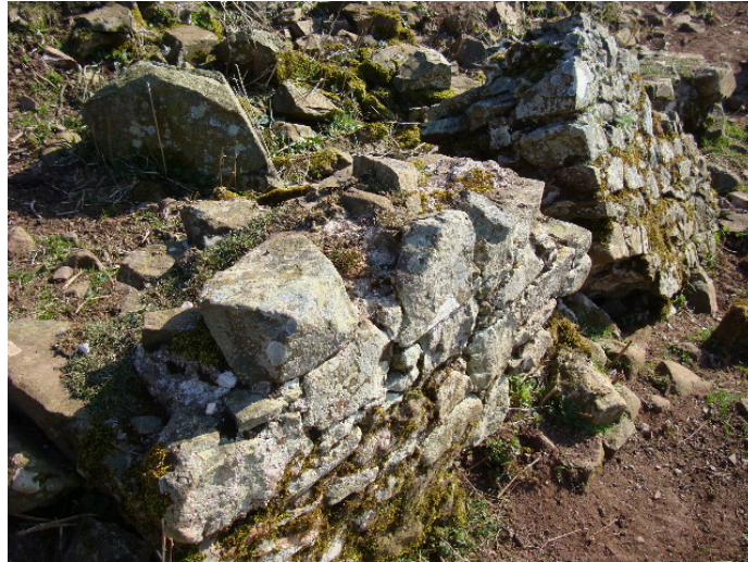
Part of structure in the mill area
