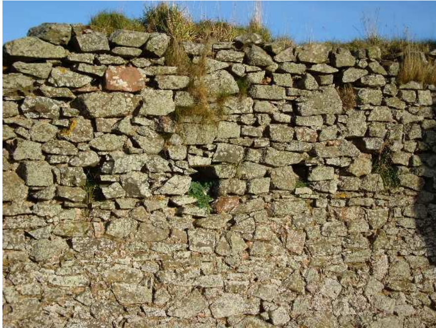
Beam slots in Improvement era house wall
