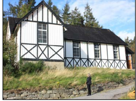
Fig 14. Milton Community Hall
