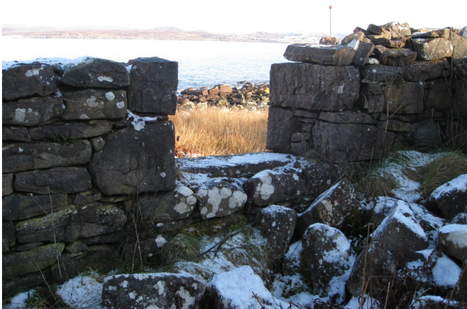
WINDOW ON N FACING SIDE OF HOUSE.
