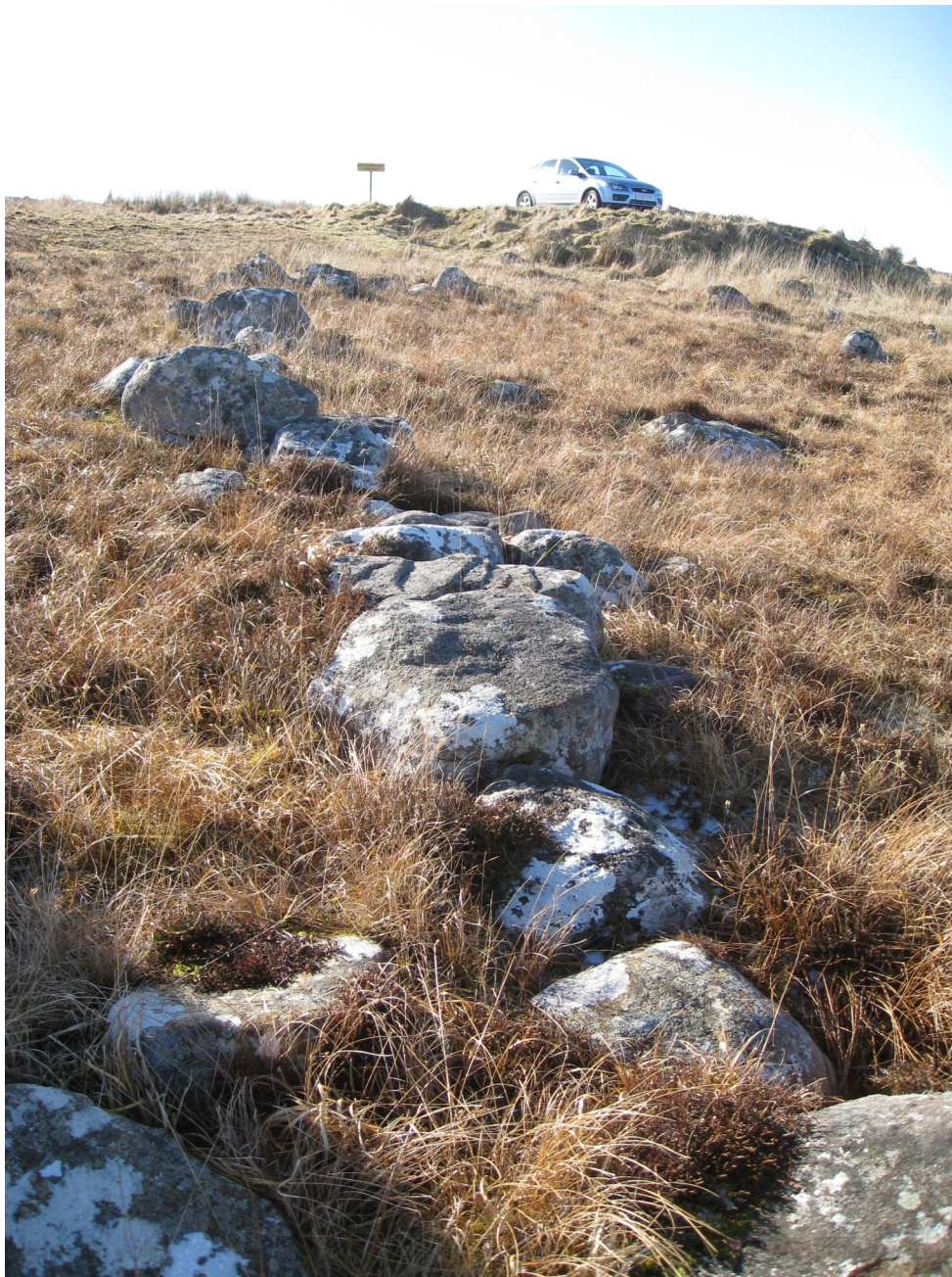
Ruinous stone dyke running down the slope on croft 1
