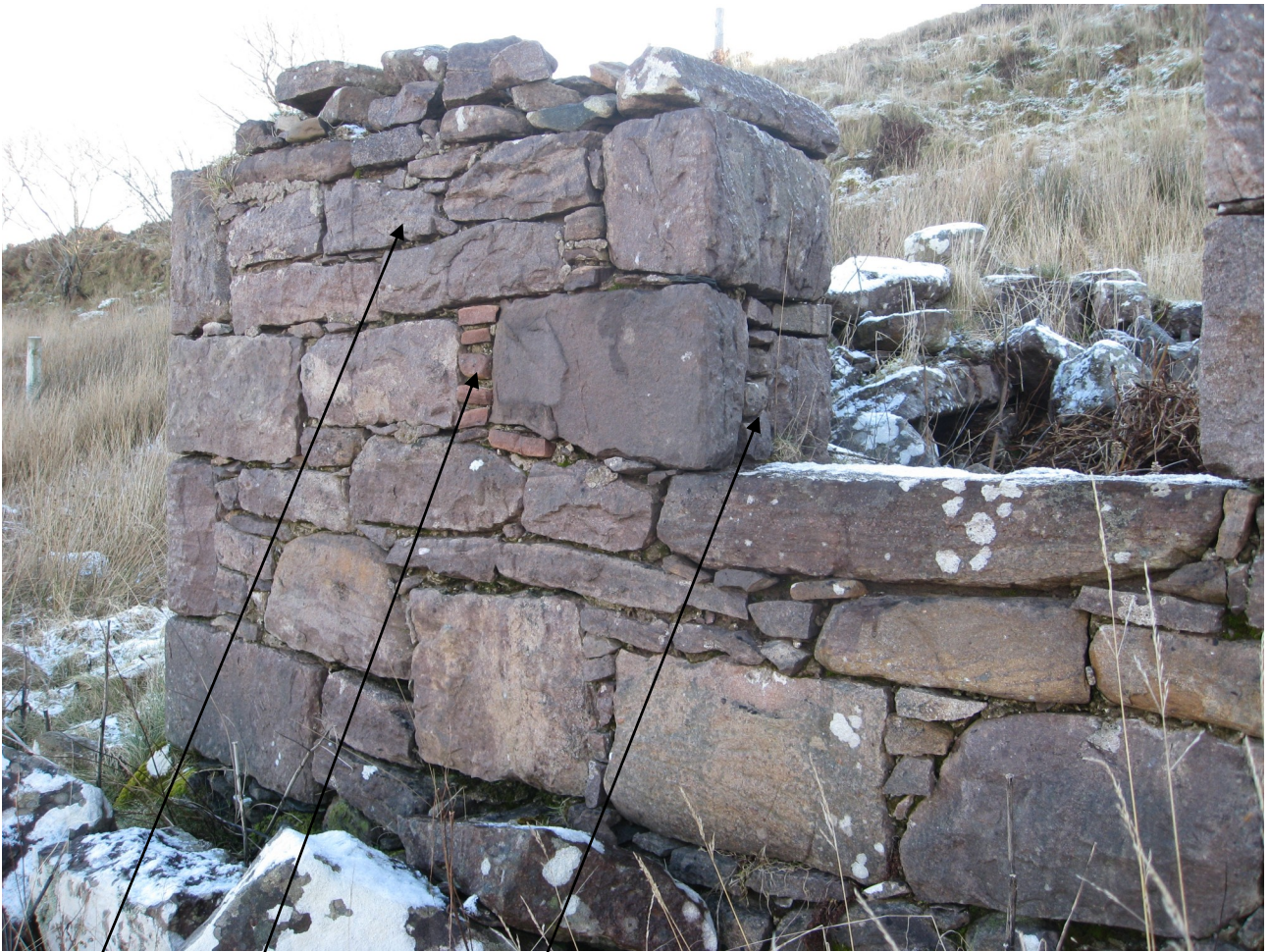
LAYERING SNECKING SLOPING SIDES OF WINDOWS
