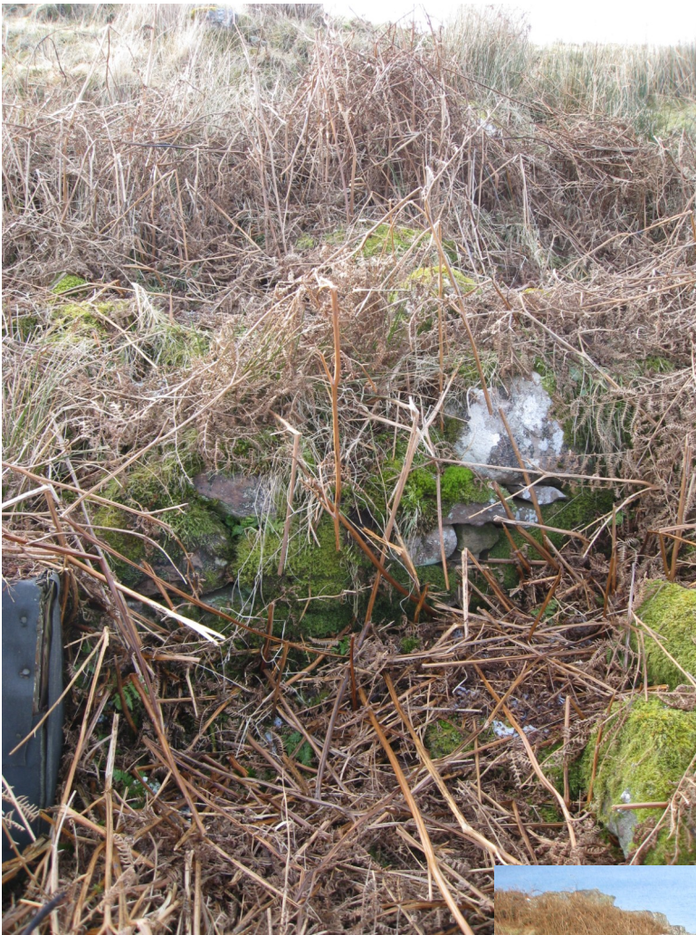
DETAIL OF W WALL BUILT INTO SLOPE OF RAISED BEACH
