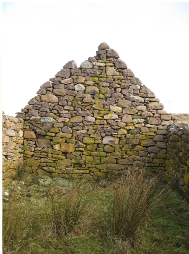
LOOKING E AT GABLE WALL
