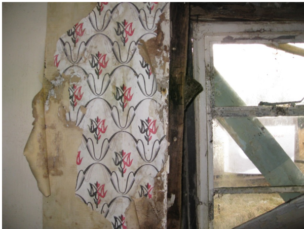
WALLPAPER BESIDE WINDOW
