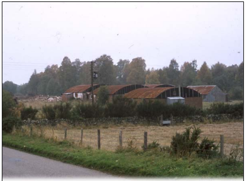
Figure 2 - Tin City Dormitory being Demolished (Source unknown, dated 16 Oct 1977)
