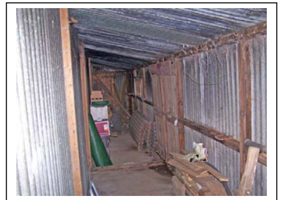
Figure 9 - Dormitory TC-19 north-side Lean-to. Internal view. (Peet 2011) Looking west
