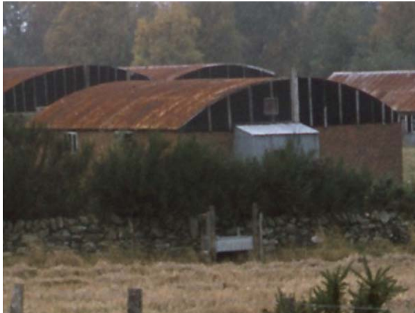
Figure 13 - Close of Tin City Dormitory (source unknown, c1977)
