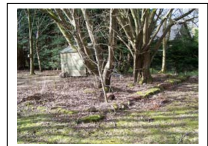
Figure 4 –Dormitory/Kitchen Foundation Remains (Peet 2008) Ref Structure TC-15; Remains W-05; Looking south-west
