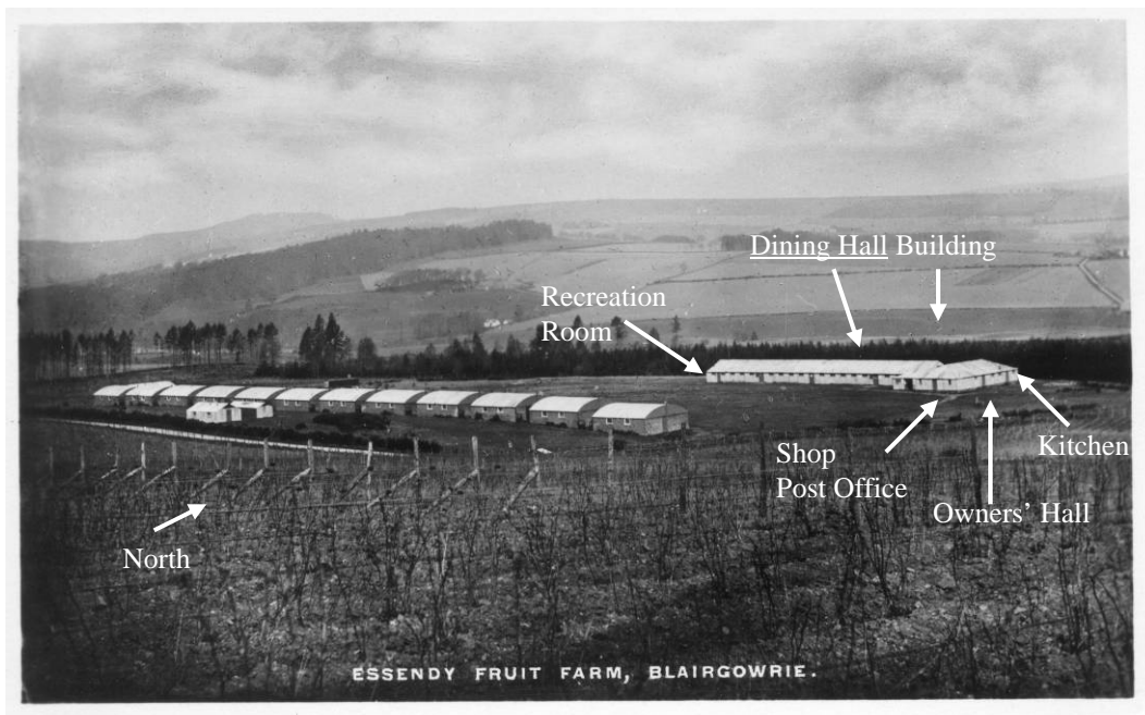
Figure 1 - Tin City Dining Hall – Location (Photo# source unknown)
