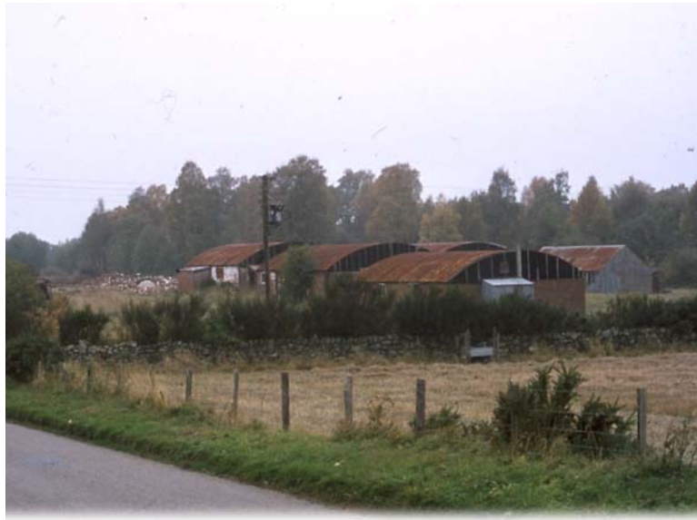
Figure 14 - Tin City Demolition 16 Oct 1977 (Source unknown)
