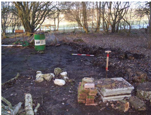
Figure 5 - Concrete Foundation W-18 (Peet 2011) Looking north
