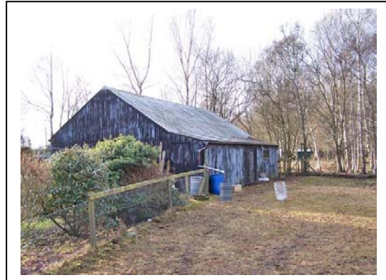
Figure 7 - Tin City Dormitory (TC-19) North and East faces (Peet 2011) Looking south-west
