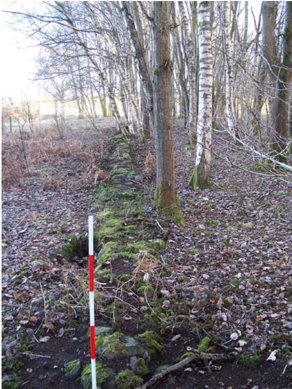
Figure 8 - Remains of Dining Hall North-side Foundation Wall (Peet 2011) Looking east
