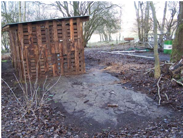
Figure 4 - Concrete Foundation W-19 (Peet 2011) Looking north
