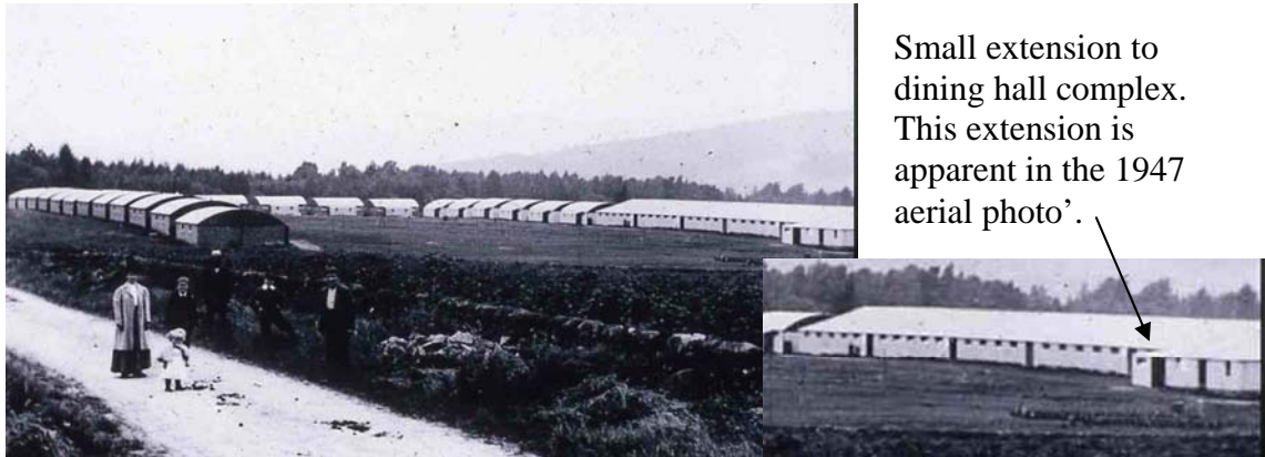
Figure 4 - Dining hall with Small Extension (Source unknown)
