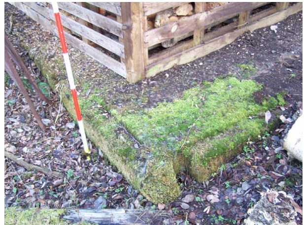
Figure 3 - Concrete Foundation W-19 - Edge Shaping for Walls (Peet 2011) North-west corner; looking ESE
