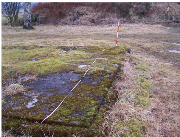
Figure 7 - Concrete Foundation W-12 (Peet 2011) Eastern end of slab; looking north
