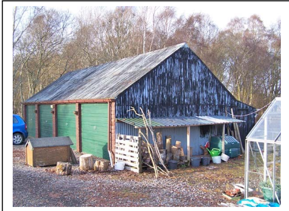
Figure 8 - Tin City Dormitory (TC-19) South and East Faces (Peet 2011) Looking north-west
