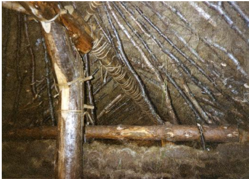
Roof detail showing a jointed cruck, roof spars and purlins with turf divots on top. Highland Folk Park 1999
