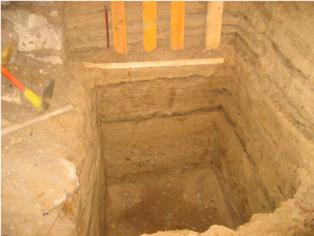
Fig. 3 - Foundation trench of retaining structure
