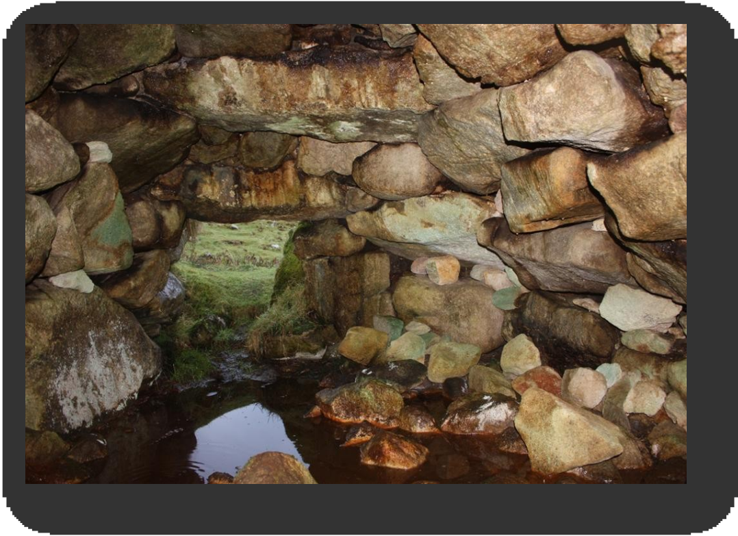
Figure 12 The whiter and small stones on the left and right have been introduced, probably since 1950. The smaller stones along the right hand side at floor level have also been introduced. Notice also the lintel at the doorway, and the way the roof lintels step up, alternating longitudinal and transverse slabs. 1148-349
