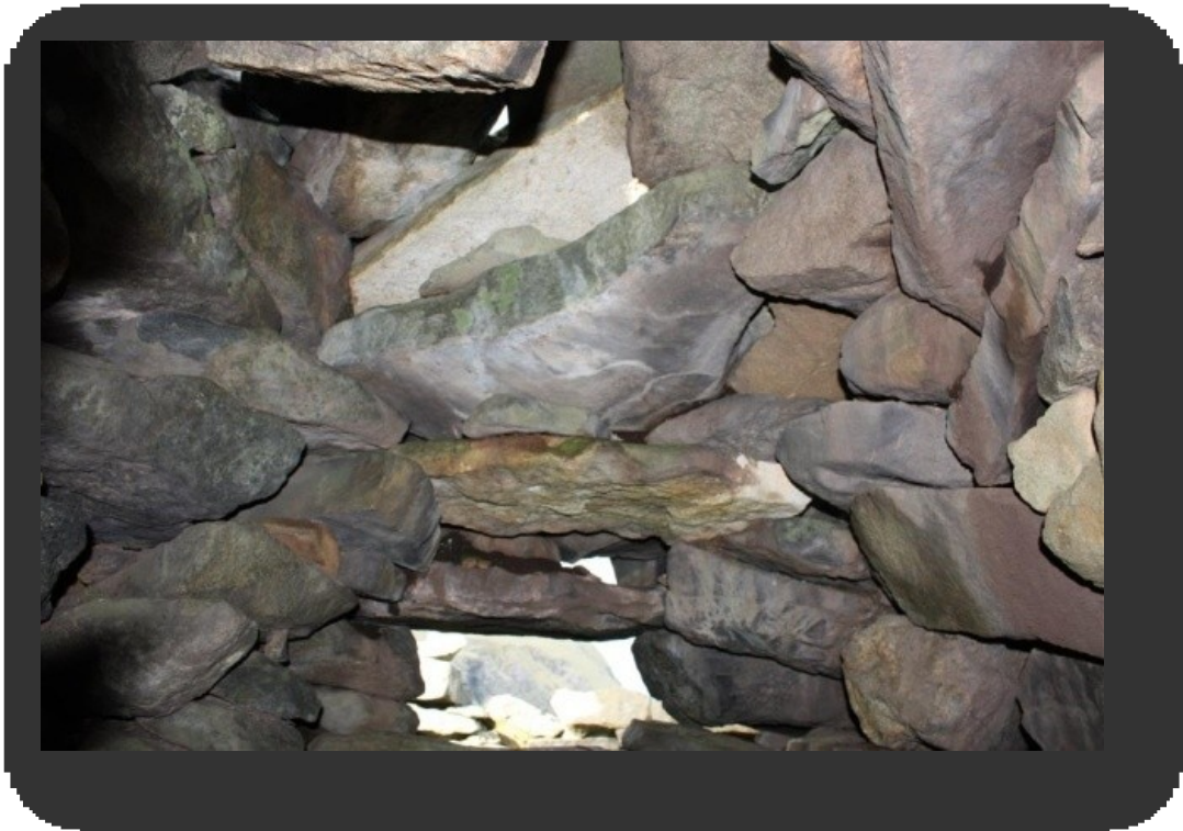
Figure 13 Two photos of the roofing slabs of the Amazon's House . In general, though irregular, they are laid 'across' the building, though three in the lower are laid 'along' the building, in this case, supported edge on edge. 1148-110 (top) and 99 (below).
