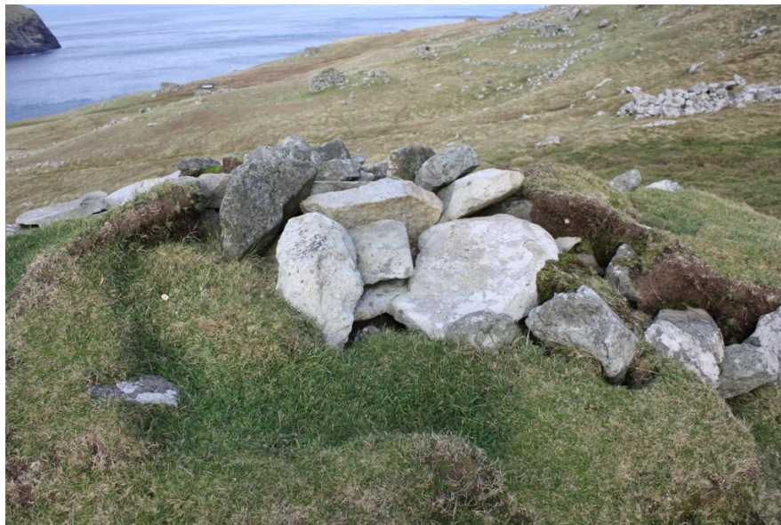
Figure 16 The roof of the Amazon's House cell. This area should be re-turfed. View from S. 1148-115 © RCAHMS.
