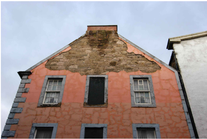
Plate 3 - South-facing elevation showing area where harling has been removed
