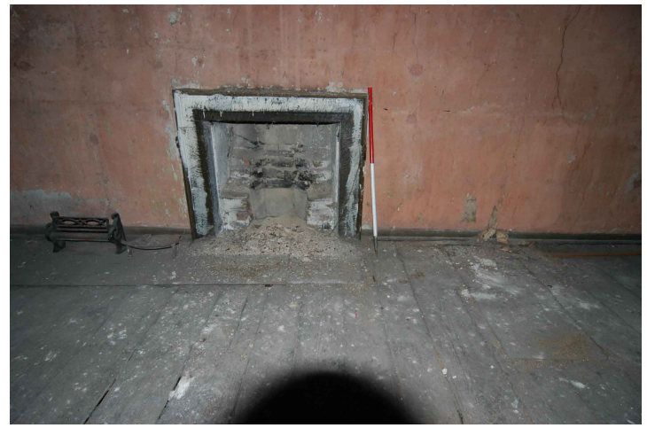
Plate 8 - Unit 18m attic room fireplace
