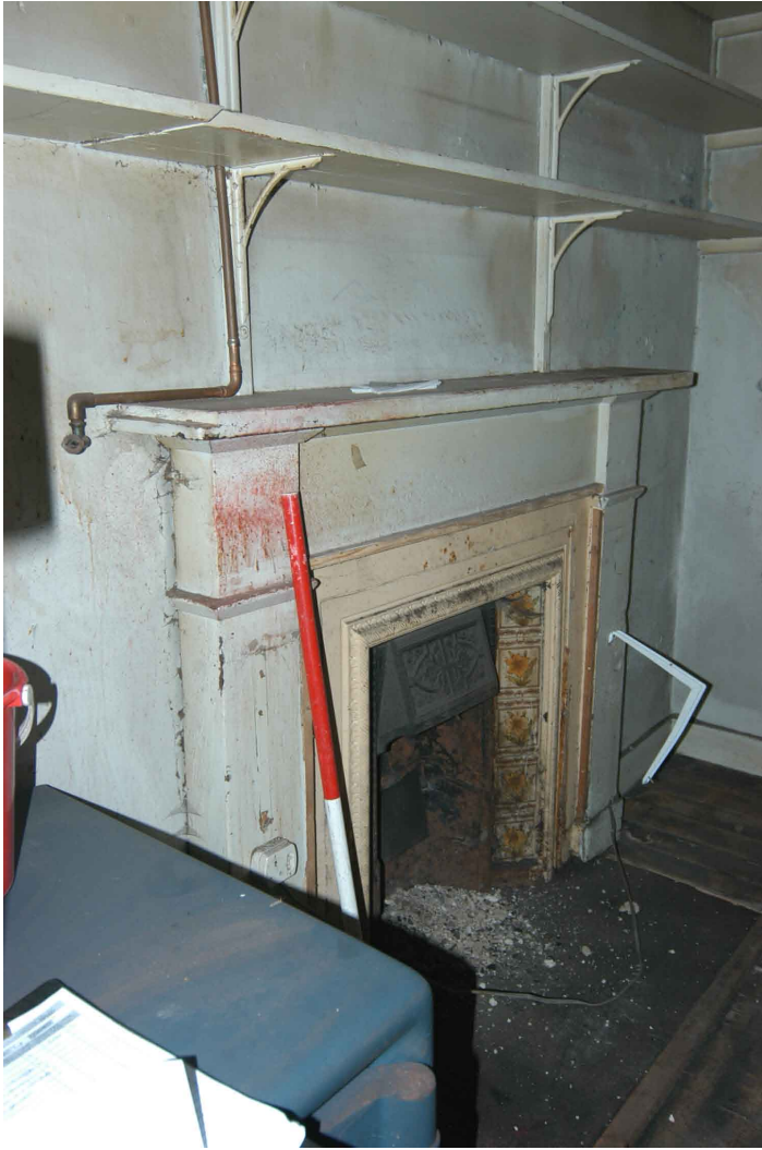
Plate 6 - Unit 6 Rear shop fireplace on the south wall
