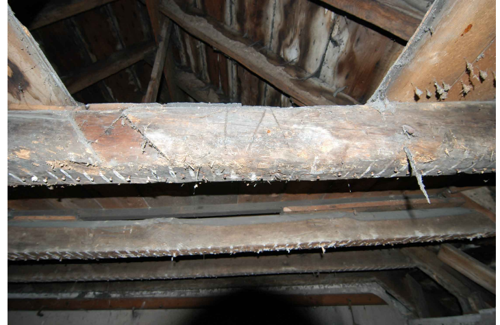
Plate 10 - Evidence of re-use of a tie beam in Unit 19 attic
