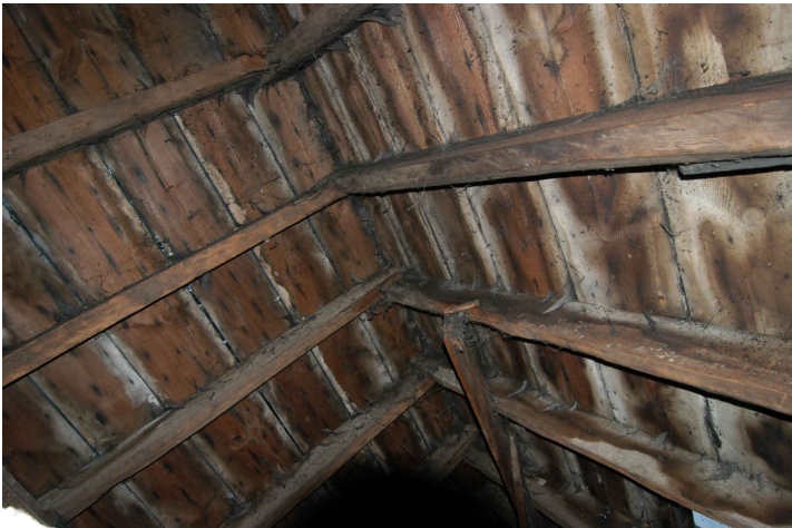
Plate 9 - A-frame roof joists and sarking
