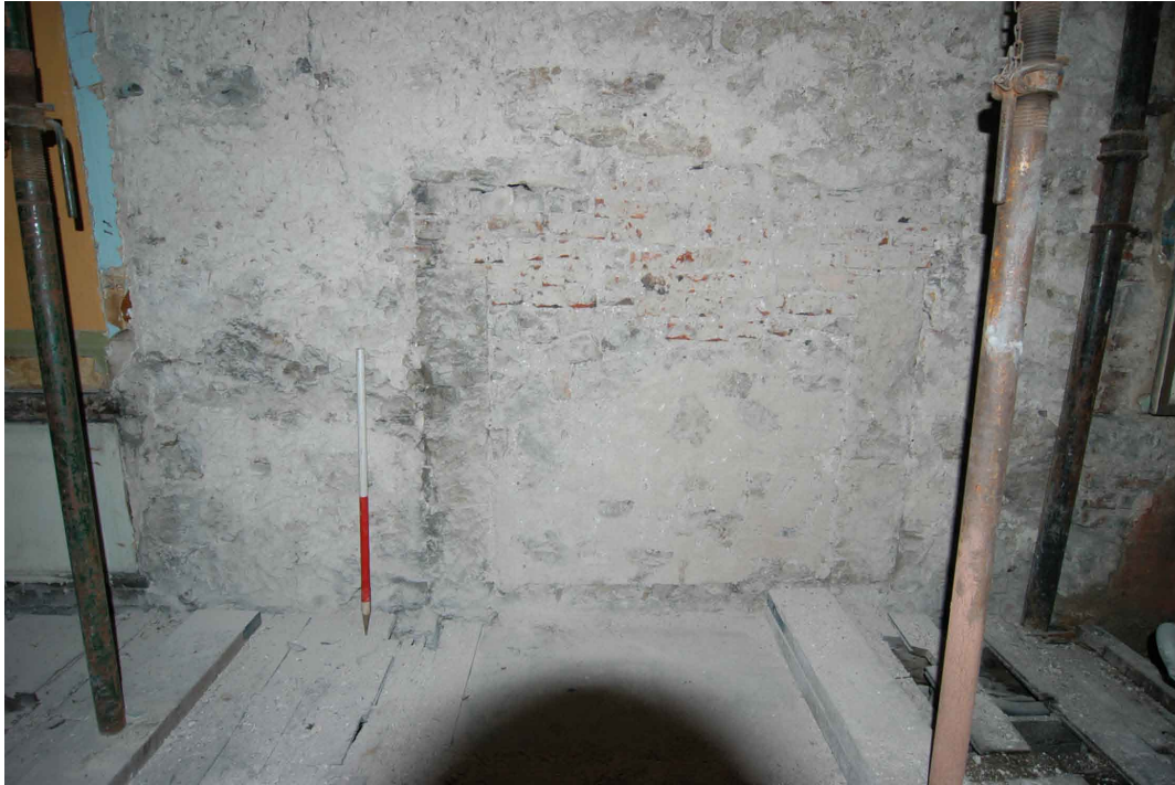
Plate 23 - Unit 9, South-facing elevation, remains of an 18th-century fireplace
