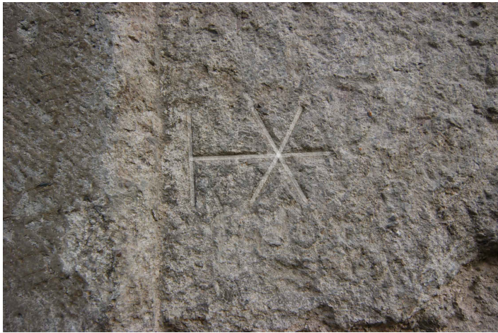
Plate 14 - The most common form of mason's mark
