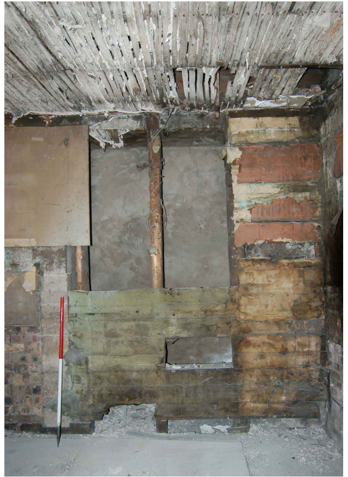
Plate 19 - Unit 1, south-facing elevation with stud panelling to the right of the fireplace
