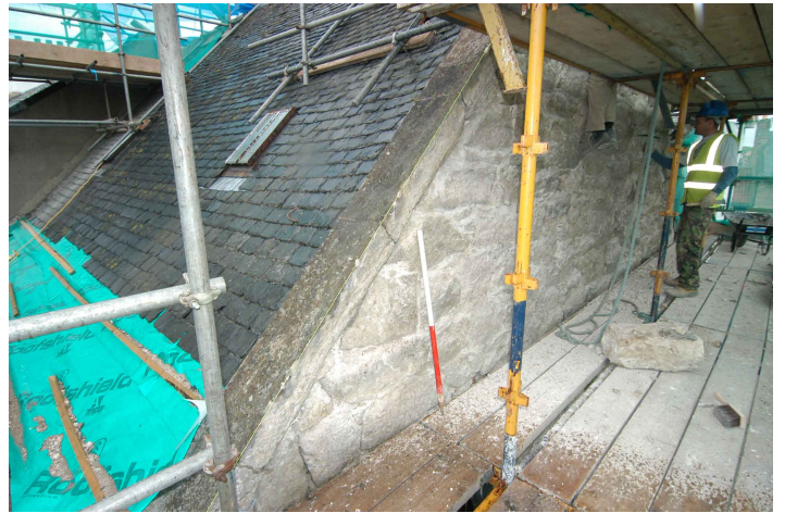
Plate 15 - Stone skew copings on the south-facing gable
