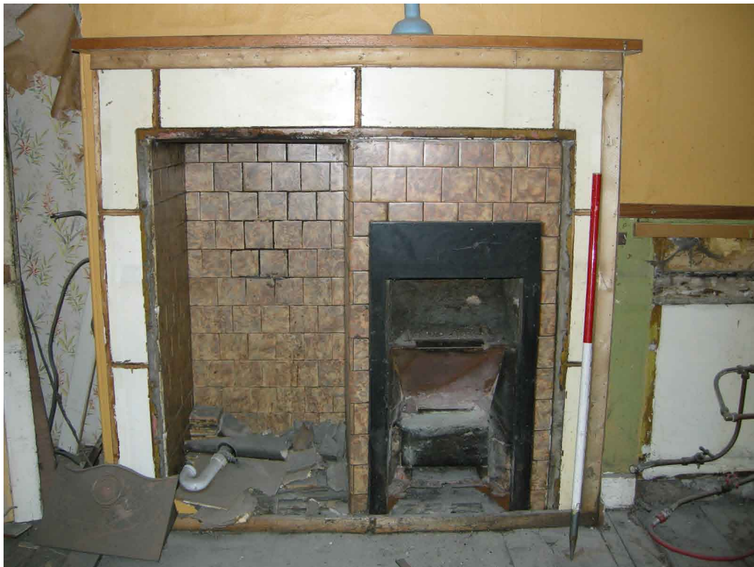
Plate 24 - Unit 11, South-facing elevation, 1950s style fireplace
