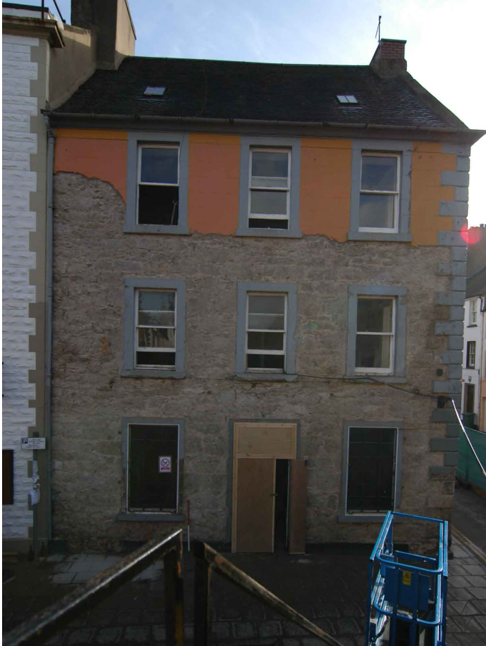
Plate 11 - West-facing elevation with harling removed to below the second floor
