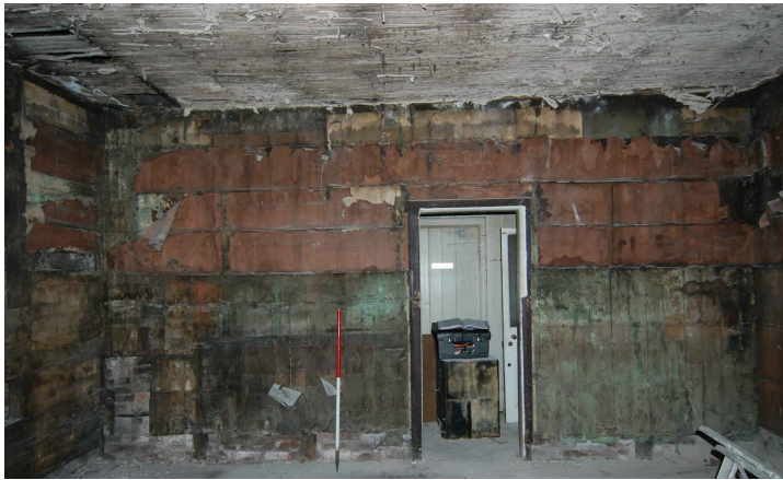
Plate 20 - Unit 1, west-facing elevation showing different wall paper and shelving scars
