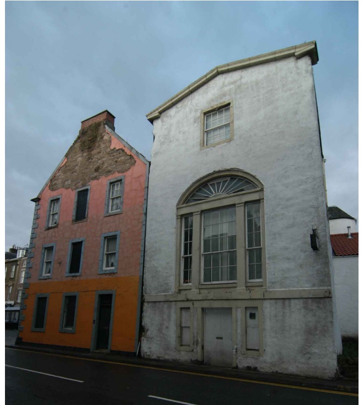
Plate 2 - South-facing elevation and the George Hotel SW extension (1822)
