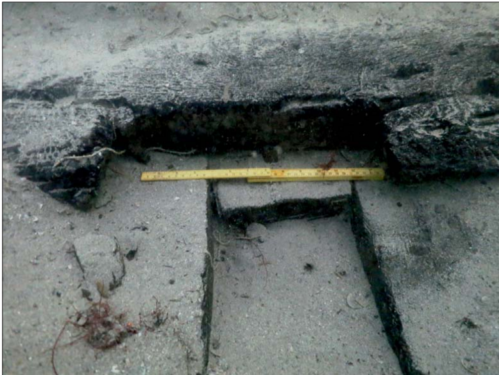
Plate 11: Section of timber framing
