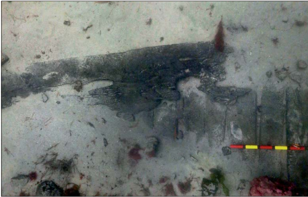
Plate 10: Photograph of ceiling timber framing showing damage by shipworm
