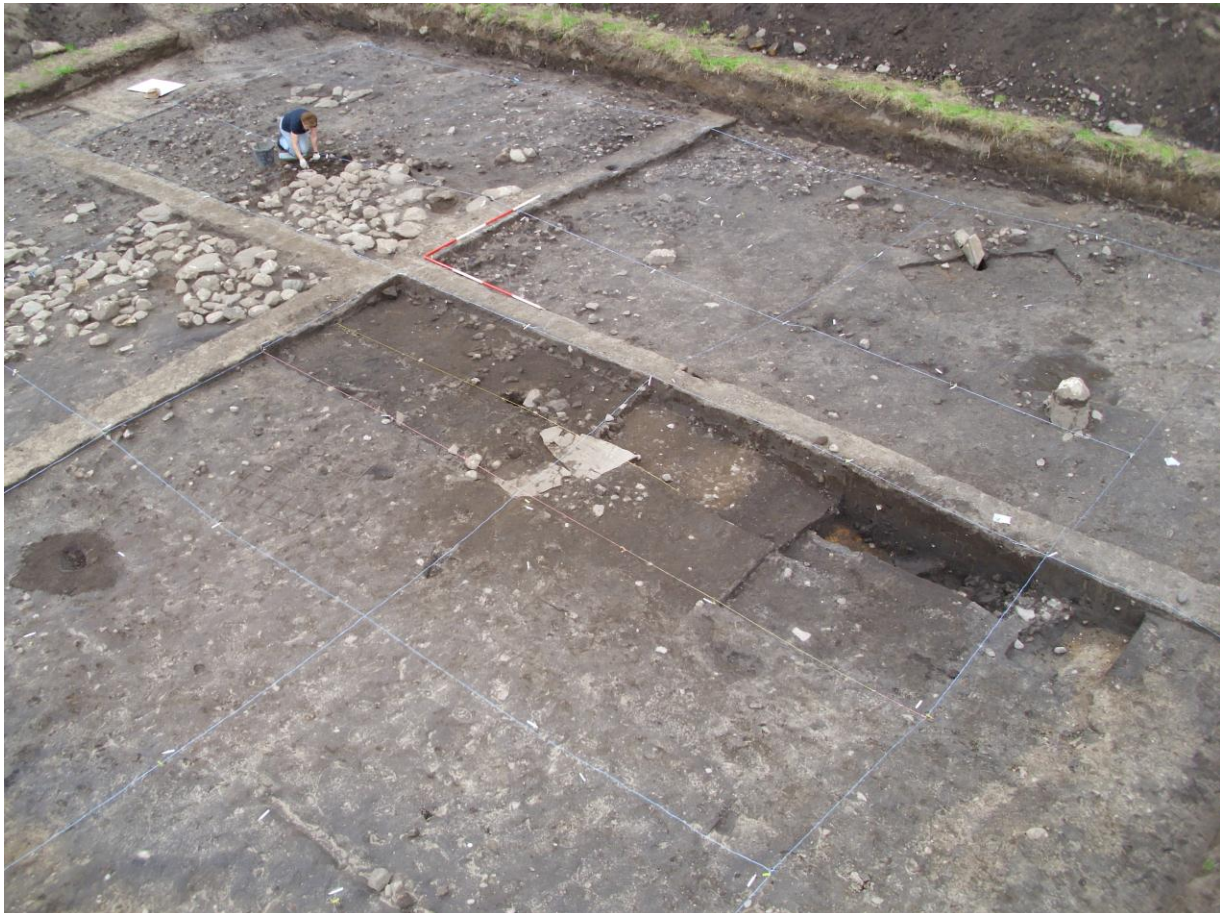
Fig 8: excavations in progress in trench B
