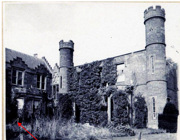
b) Photograph - 1956 RCAHMS AN1571-8 View from SW
