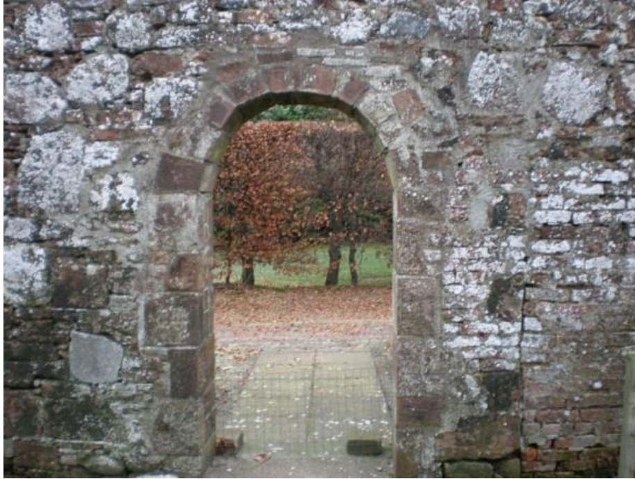
Arched Exit Doorway on North East Wall
