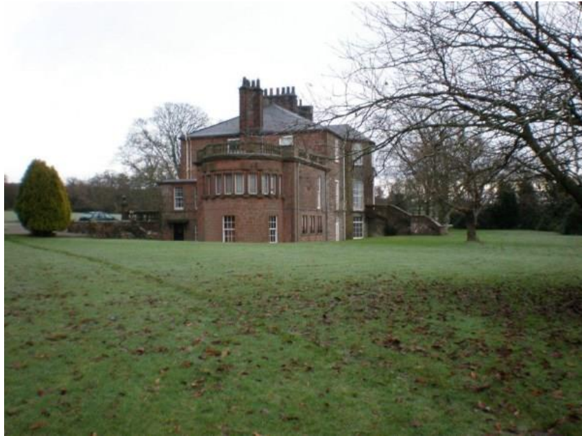
Conheath House: South East Aspect From Walled Garden
