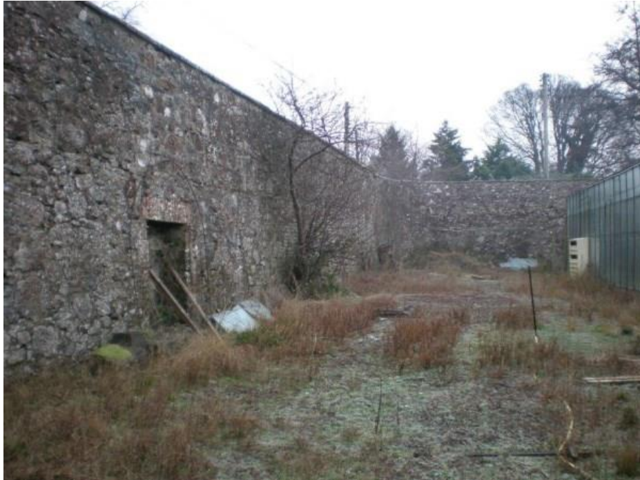
Curved North East Corner of Garden Wall
