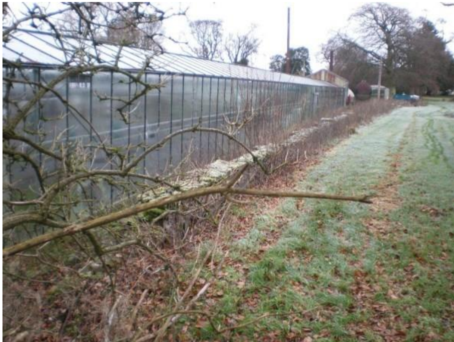
Exterior of Low South East Wall
