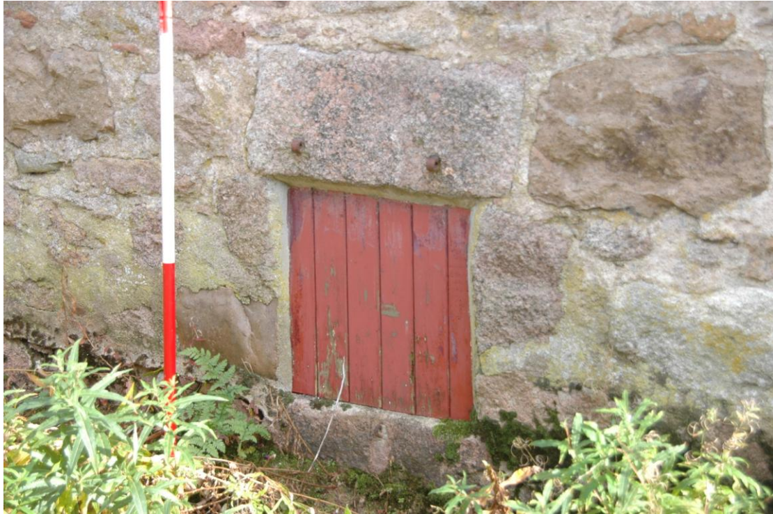
Illus 21 Vent 2 in the W wall showing pivots for original shutter and later wooden blocking.
