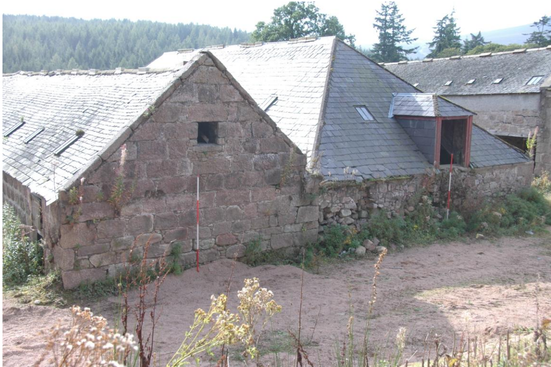
Illus 20 N side of building 2 with older part to LHS and the difference in walling clear between it and the W part on the RHS
