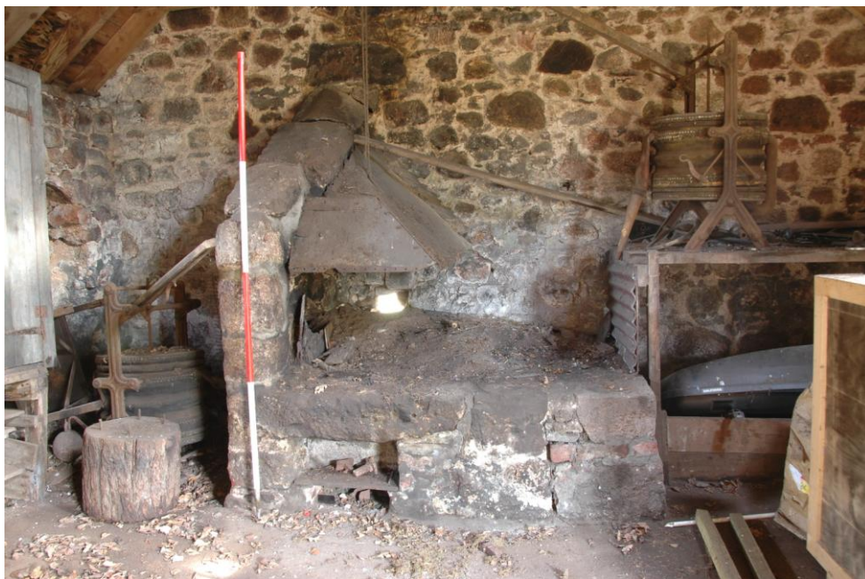
Illus 27 Forge - vent can be seen above forge bed
