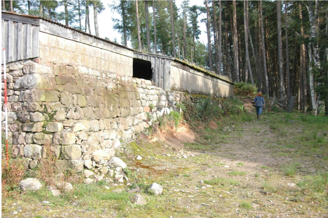
Illus 33 S side of buildings 4 and 5 showing the earlier revetting wall
