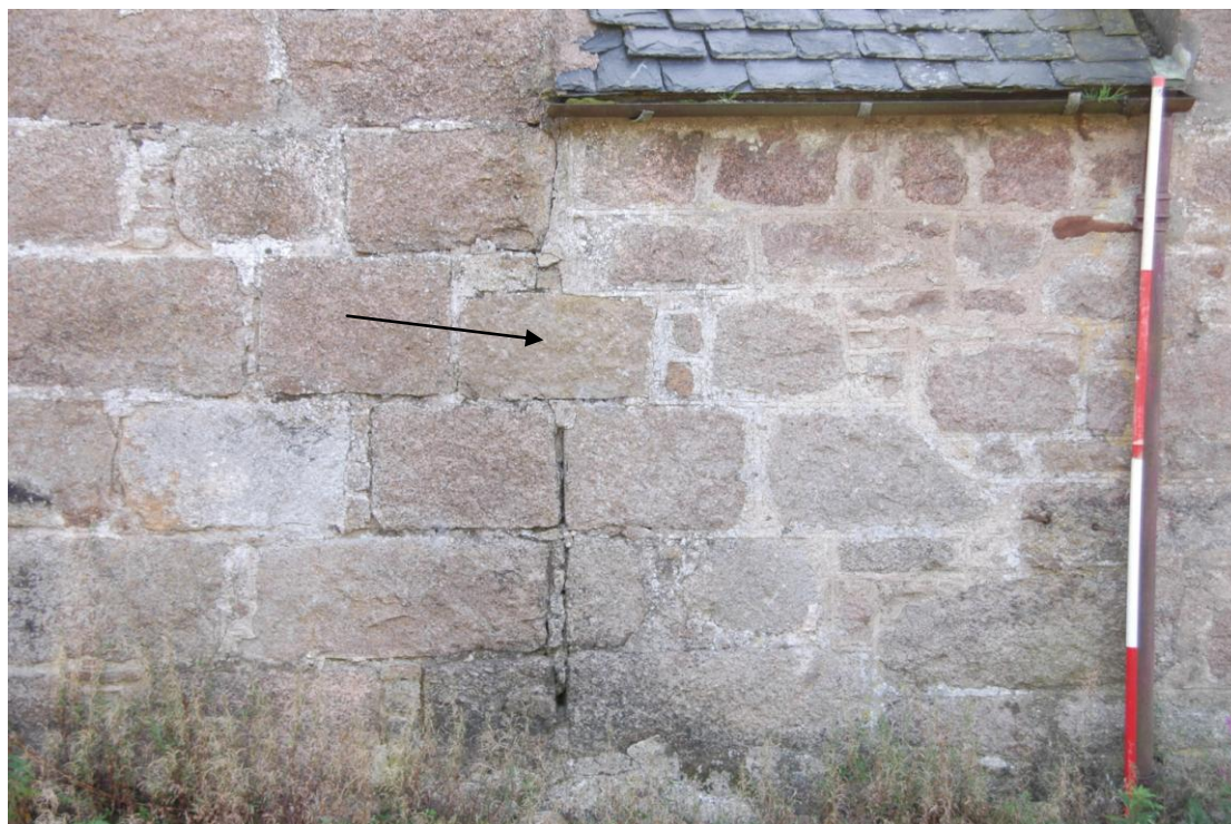
Illus 11 Building 1 wall 1a and 1b showing different stonework
