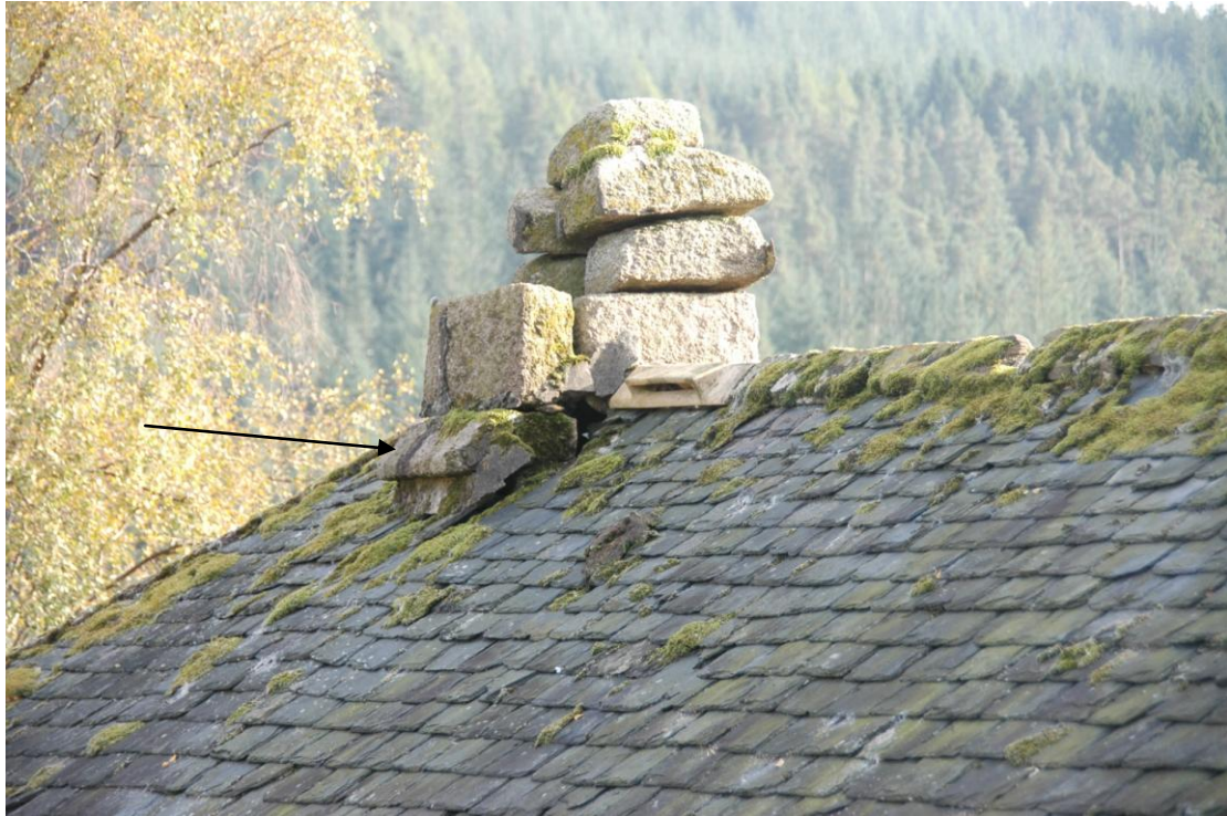
Illus 36 Chimney in Building 6 showing ledge which suggests thatch
