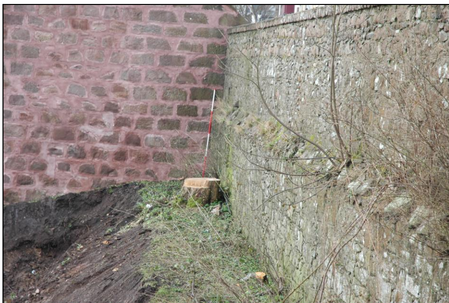
Illus. 9: Inner face of boundary wall and revetting wall.
