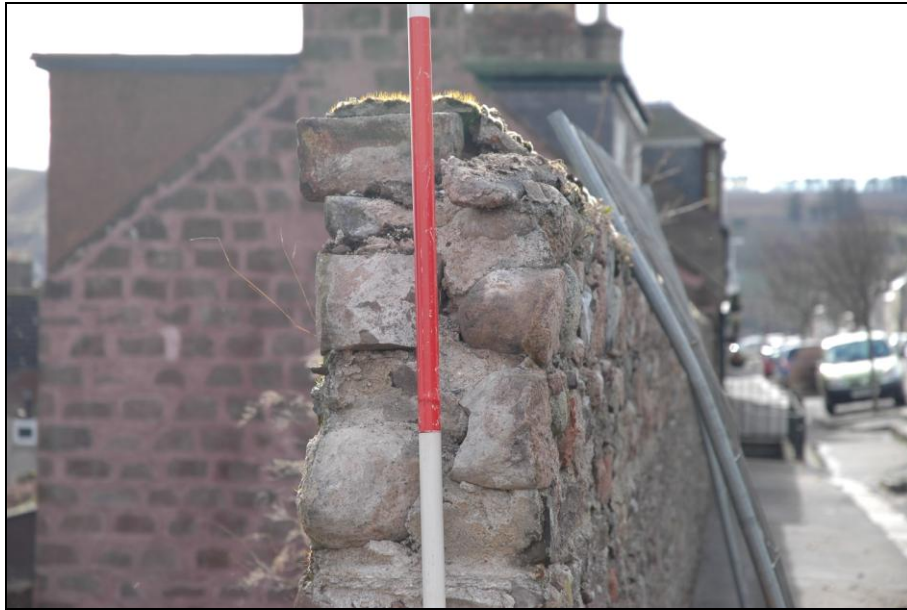
Illus. 8: View, S, of the wall construction.
