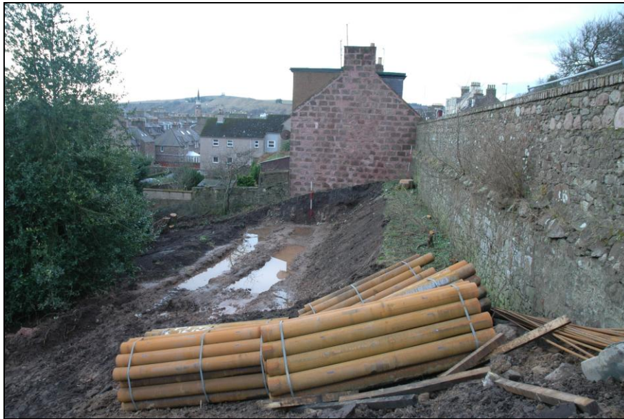
Illus. 4: View, S, of SW sector of the site.
