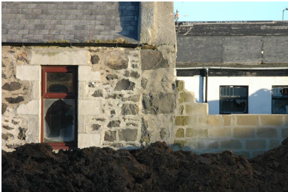
Illus 4 South end of back (west) wall of Building 2 showing double thickness of gable Walls to the south of building 2. The line of the front wall of the cottage was continued to the south by a low stone wall foundation, 600mm wide (Illus 2: Wall 1).
