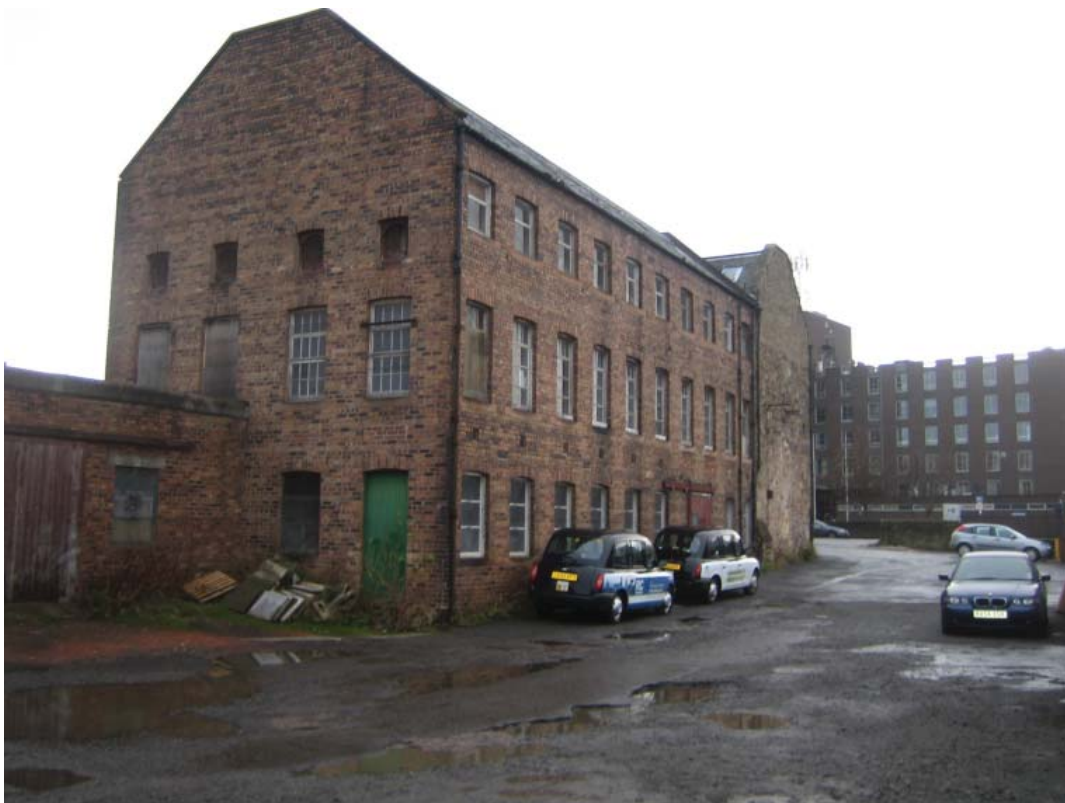
Plate 2: Brick extension to rear of mill showing current ground surface
