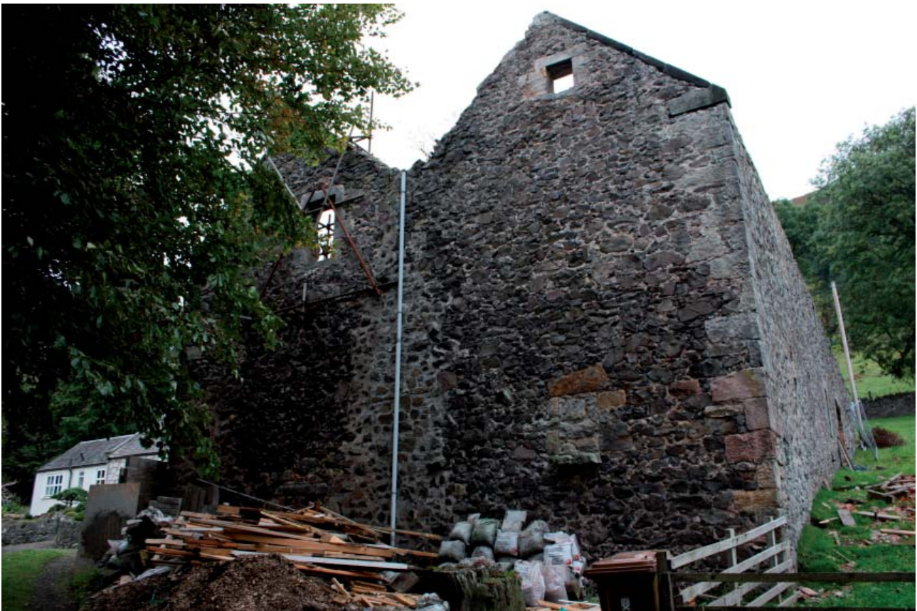
Illus 5 View of south wall (from the south)
