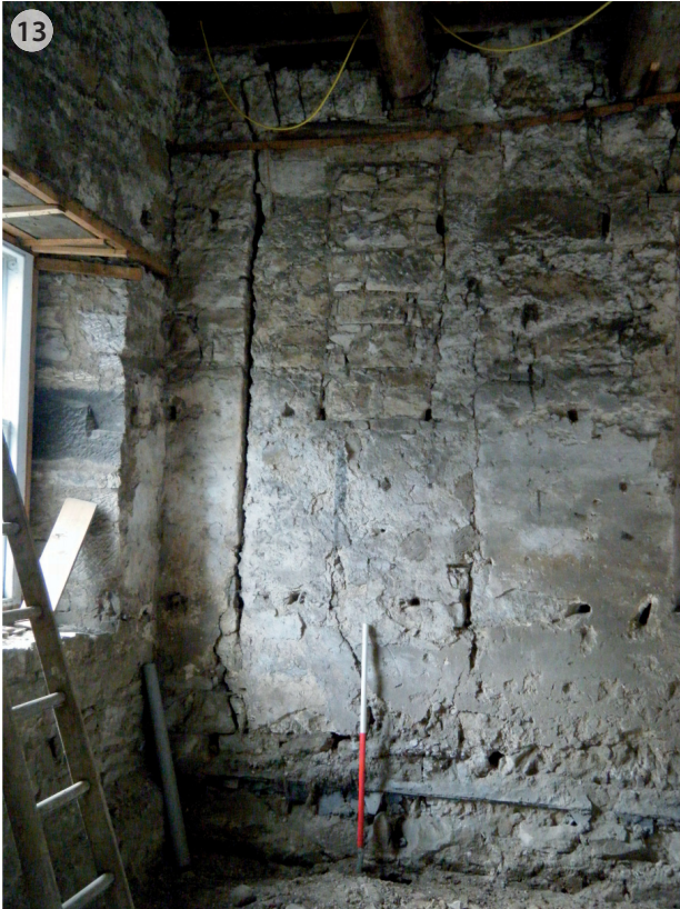
Illus 13 Internal view of stone-blocked feature GW17
