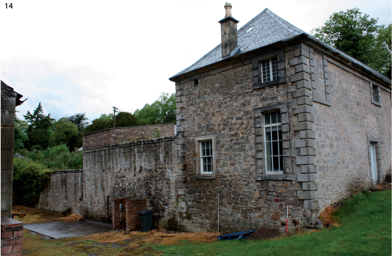
Illus 14 General view of the external south elevation
