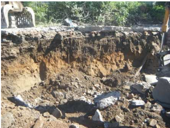
Illus 6 General view of the north facing section showing the geological sand layer (003) below the topsoil
