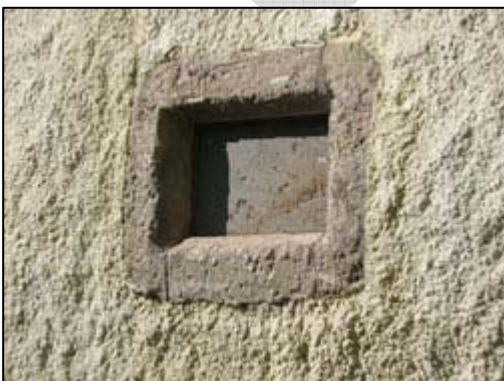
Fig. 2g: Blocking of Window
