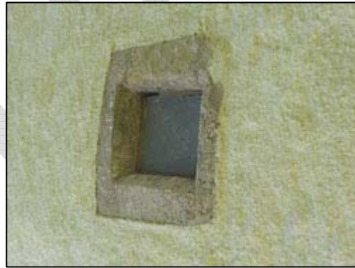
Fig. 2f: Blocking of Window
