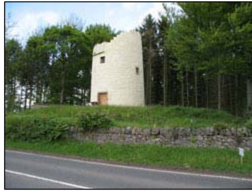
Fig. 2b: From the South-east
