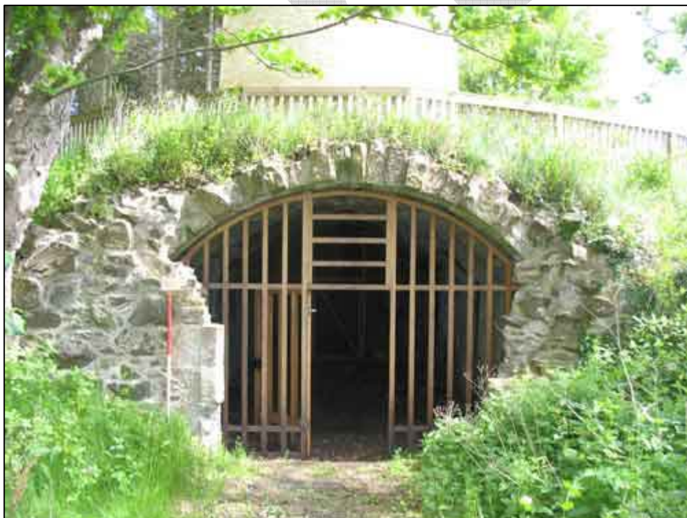
Fig. 3b: View Showing Entrance to Vaulted Chamber
