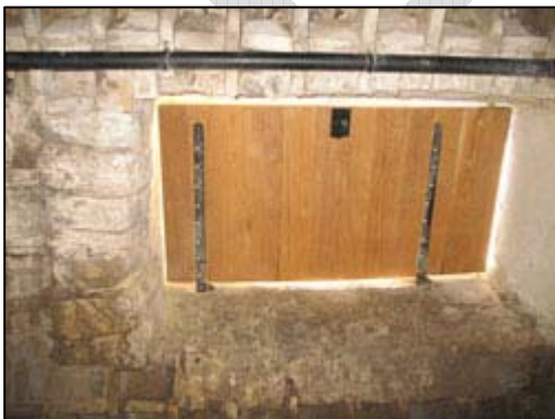
Fig. 4g: Interior view of doorway
