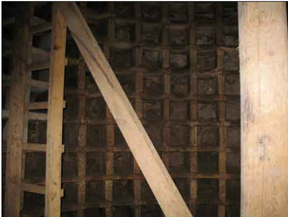
Fig. 3a: Interior View, Showing Nestboxes and Potence
