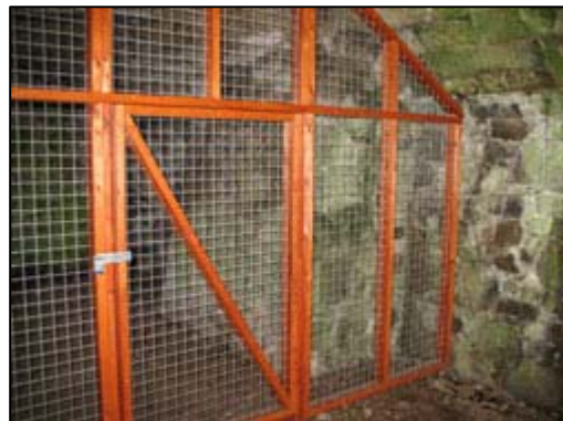
Fig. 4h: Modern partition in vault
