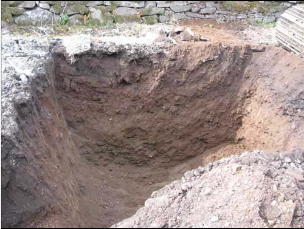
Fig. 4a: Area 1 (Farmyard): Pit for Septic Tank
