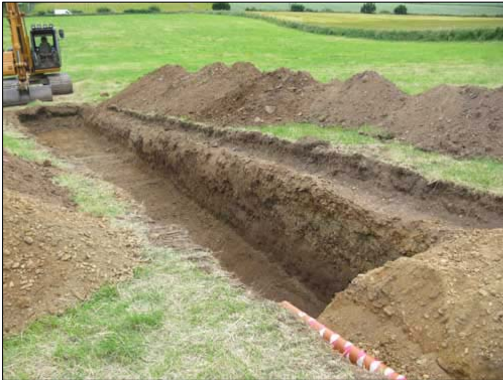
Fig. 5a: Area 2 (Field) : Footprint of Soakaway, Topsoil stripped.
