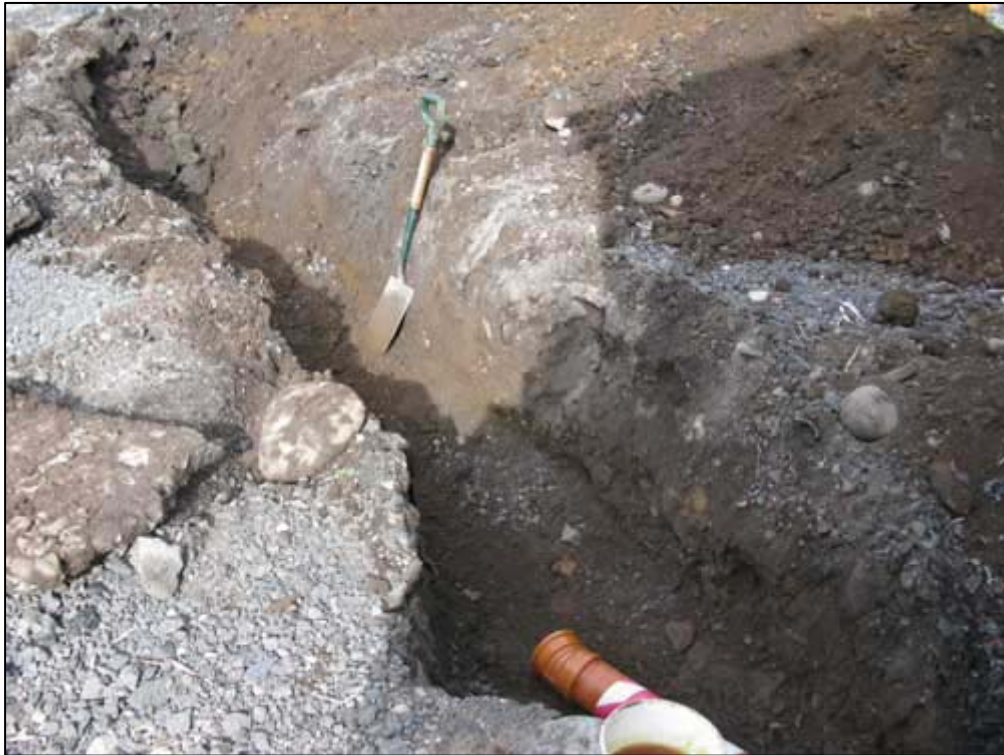
Fig. 3b: Area 1 (Farmyard): Drainage Track, Post-Excavation
