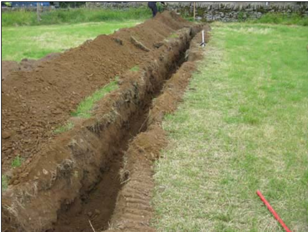
Fig. 4a: Area 1 (Farmyard): Pit for Septic Tank
