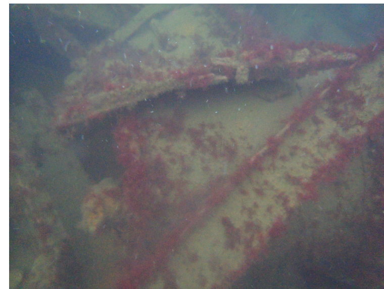
Miscellaneous hull plating
