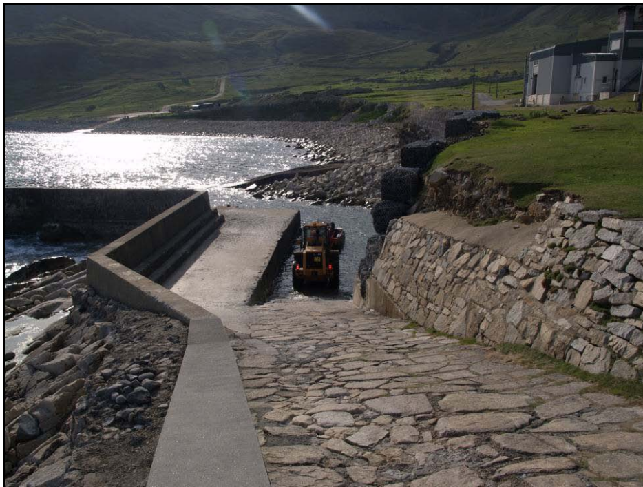
The modern pier from the north east during 2008. The wheel loader is used to launch the rigid inflatable used by the radar base. The position of the original pier is visible in the parapet wall and as a faint line in the main concrete platform.
