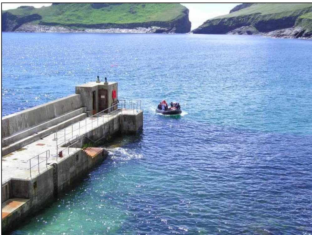
Visitors approaching the modern pier during the summer of 2008. The building at the end of the pier is the pump house.
