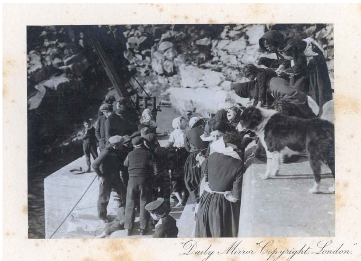
A historic photograph from 1912 showing a busy day on the pier, probably just after the arrival of a steamer. The 15 tonne crane and mooring rings are visible and the steps have already been damaged by boulders thrown by the sea. © Museum nan Eilean, Western Isles Council
