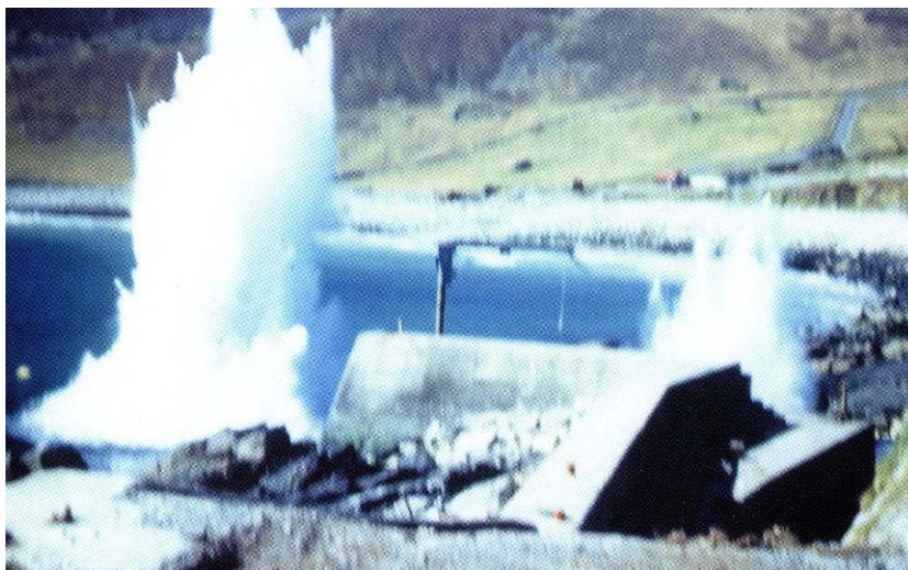
The pier from the east during blasting to clear boulders in the late 1950s (Mackay 2002)
