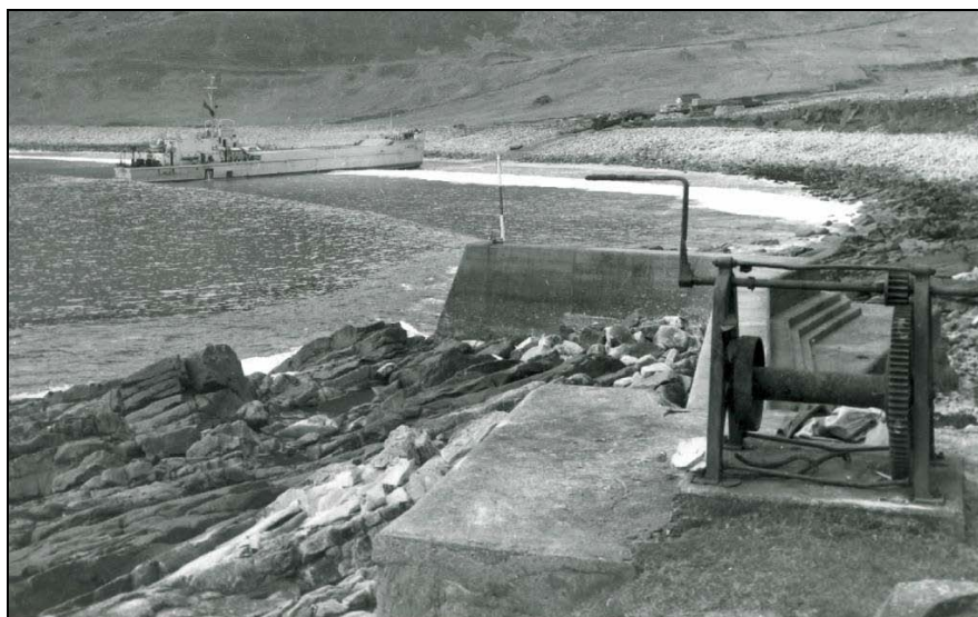
The pier from the south east in the late 1950s or early 1960s showing the new winch installed by Mr Monk c.1911 (SKA315)
