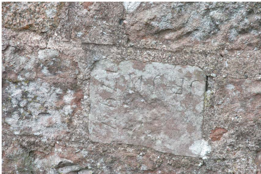
Illus 3 Bothy detail of date stone, probably reused
