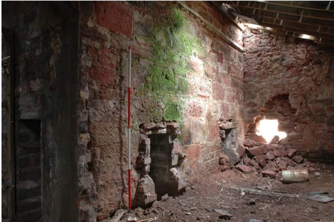
Illus 13 Steading, Area 5 detail of grain chutes broken through mill wall
