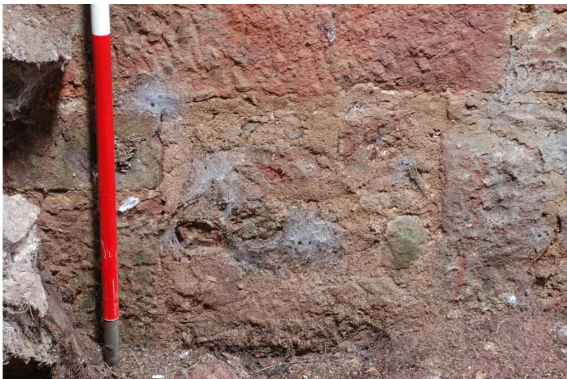
Illus 18 Mill wall showing blocked wheel shaft hole
