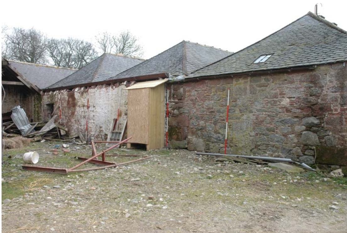
Illus 9 Steading wall 3 with ranging rods indicating vents
