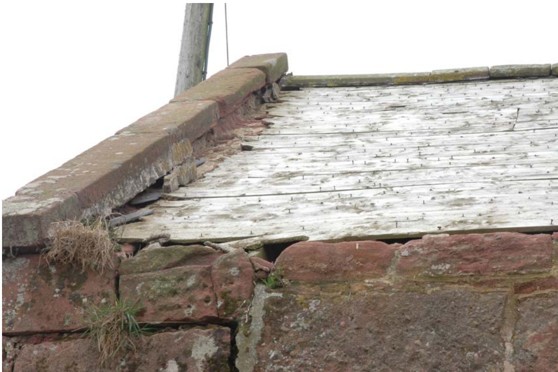
Illus 21 Mill Detail of S skew
