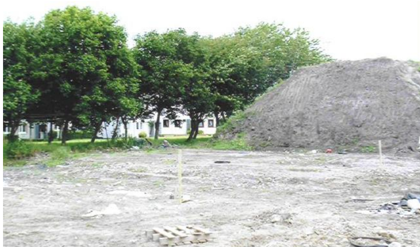
View of site before excavation facing NW
