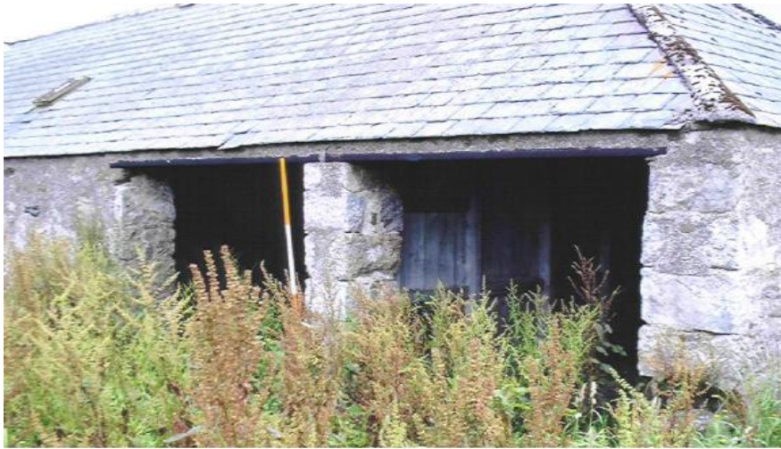
Detail of cartsheds entrance - scale 2m
