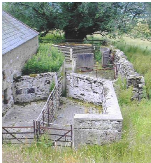
View of sheep dip and pens for rear facing SE
