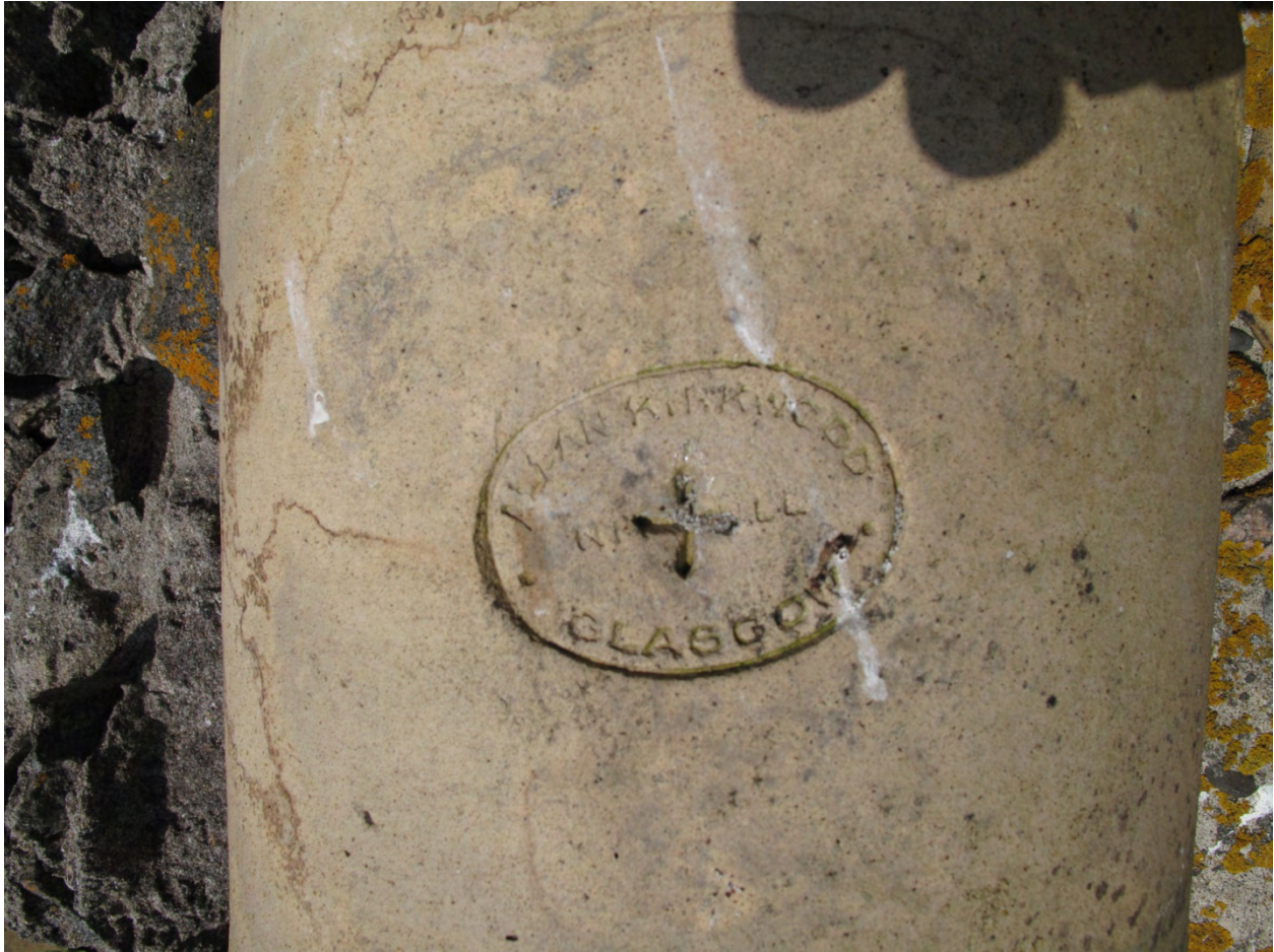
Figure 12 Detail of the stamp on a chimney can. 'Allan Kirkwood, Nitshill, Glasgow'.
