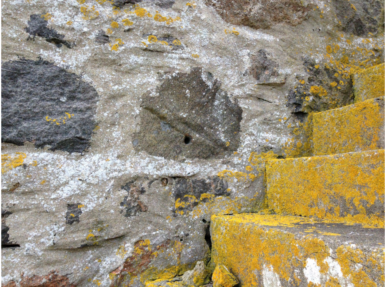
Figure 4 The stonework of granite and gneiss is 'sneck-harled' ie there is a mortar coating that covers over all the joints and pinnings (snecking) but does not extend over all the stonework. Holes created by drilling during the quarrying process (known as 'jumpers' are visible on a number of the stones. The staircase is finished in concrete, presumably over a concrete base.
