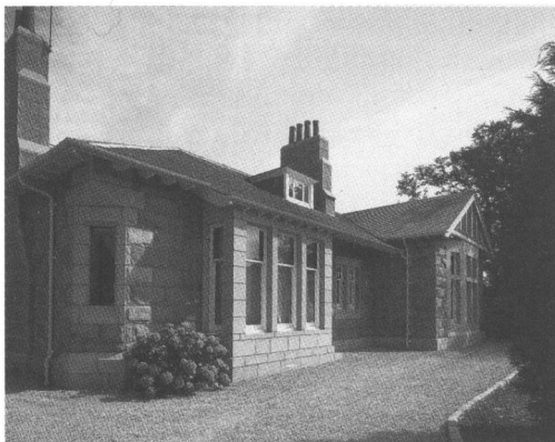
59 The Chalet, 4 Anderson Drive, 1904, by G. Fordyce: 1991 view. A more luxurious precursor of the city's ubiquitous single-storeyed interwar bungalows (RCAHMS B56421).
