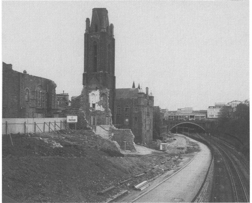
97 Construction of the Inner Ring Road in progress along the Denburn valley in 1992, with the partly demolished 'Triple Kirks' on its left (RCAHMS B70422).
