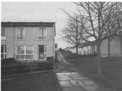
87 'The Hillocks' development, Bucksburn, 1965–8; 1992 view. A scheme of housing built by Aberdeenshire County Council (on a site which was at that time beyond the city boundaries) as a design-and-build 'package-deal' by Wimpey. The photograph shows the 'Radburn'-style segregation of pedestrian and vehicular access (RCAHMS B70442).
