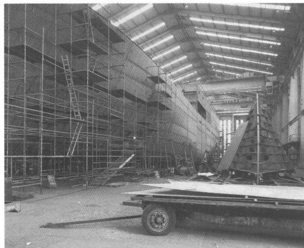
49 Hall Russell Shipyard, 1989 view along west side of building hall, showing Ship No.1000 (a welded-steel, twin-screw cargo-passenger ferry for the St Helena service) under construction (RCAHMS B17858).
