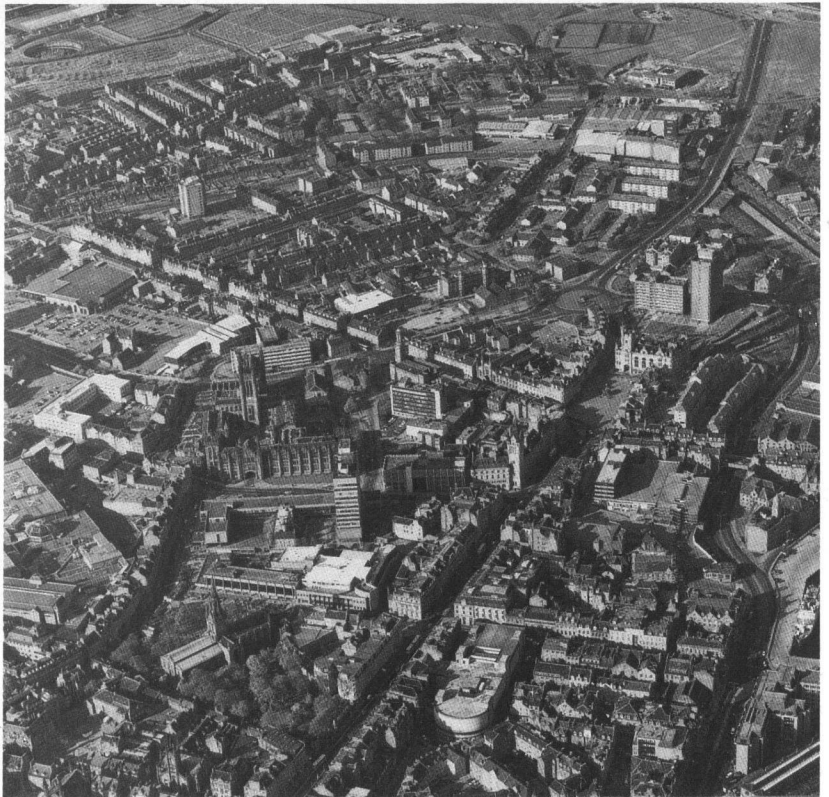
68 Aerial view (1996) of the east end of Union Street and Castlegate, showing Marischal College and the Town House complex (at centre) and the Castlehill multi-storey Corporation housing blocks of 1965-8 at upper right (RCAHMS C56412).
