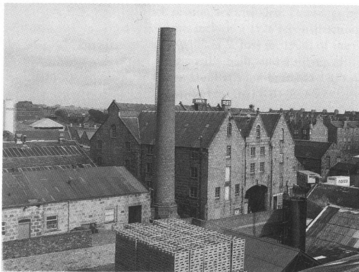
115 Millbank Mills, Berryden Road, from the south. Recorded in 1983 as part of RCAHMS industrial survey work (RCAHMS A3711).
