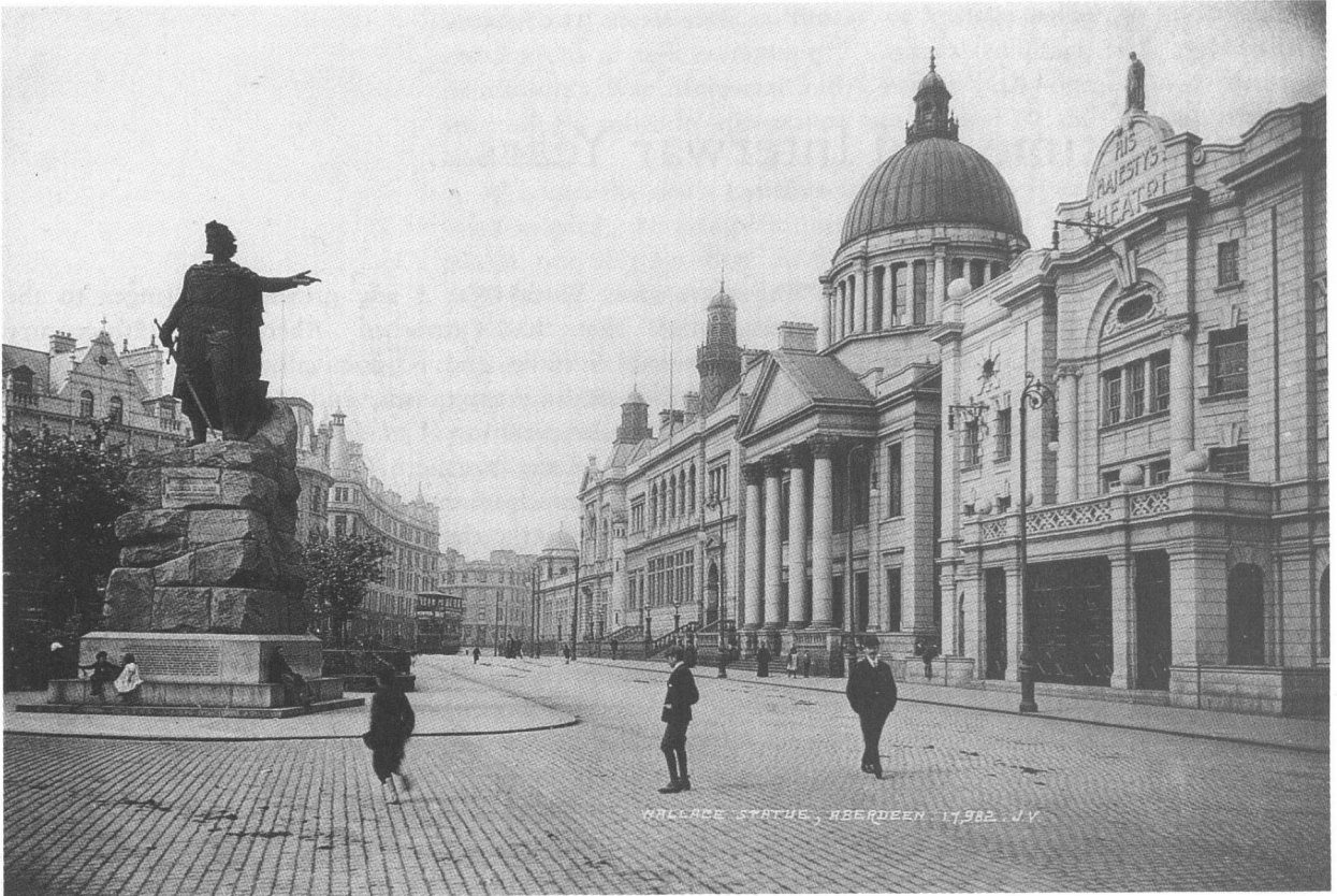
69 Rosemount Viaduct, seen in 1892 following the completion of most of the City Improvement scheme. From left to right: statue of Wallace, 1888, by W. Grant Stevenson; Public Library, 1891–2, by Brown & Watt; South United Free Church, 1892, by A. Marshall Mackenzie; His Majesty's Theatre, 1904–8, by F. Matcham (RCAHMS AB/3525).
