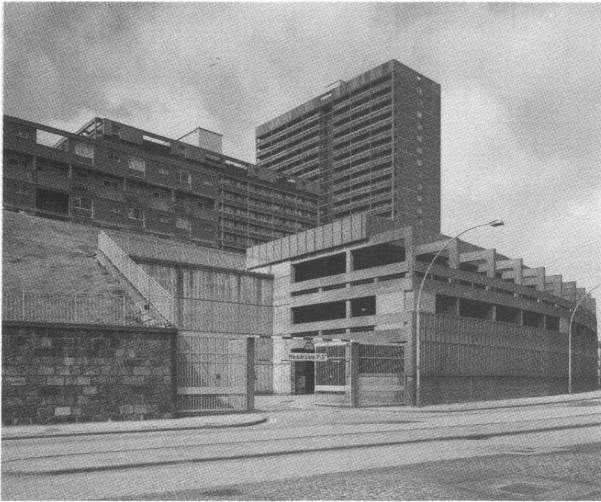
84 Gallowgate multi-storey re-development area, 1965–6, designed by the City Architect's Department; 1986 view (RCAHMS A42195).
