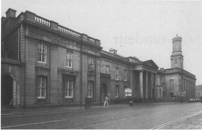
39 West side of King Street, showing (from left) John Smith's County Record Office (1832-3), Simpson's Medico-Chirurgical Hall (1818-20) and Smith's North Church (1830); 1991 view (RCAHMS B57448).
