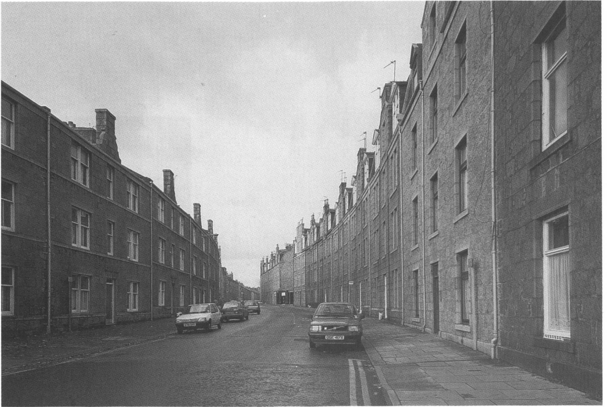
66 Urquhart Road, view of typical 1890s three- and four-storeyed granite-built tenements, showing (on the right) the ubiquitous Aberdeen top-floor mansard storey, and (on the left), Aberdeen Corporation's first housing scheme, built in 1897 (RCAHMS B55654).
