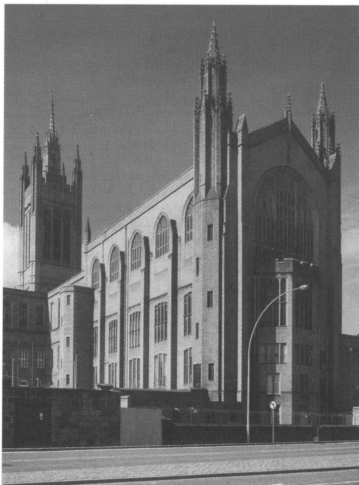
136 Marischal College Extension, 1994 view from east (RCAHMS C16708/CN).
