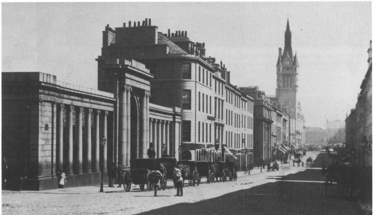
30 Late 19th-century view of Union Street from the west, showing John Smith's churchyard screen of 1829 on the left, and the new Town House in the distance (RCAHMS B13802).
