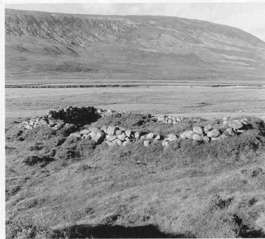
Wester Auchavrie, Glen Lui (C on maps): 18th-century farmhouse with low, random-rubble walls and rounded ends.
