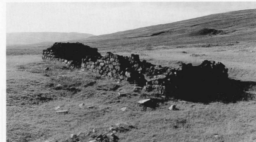
Tomnagaoithe, Glen Dee (E on maps): early 19th-century farmhouse with coursed, roughly-dressed rubble walls.
