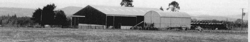
Shapark Farm, on the Black Isle, was rebuilt in 1999 by contractor John Duncan of Buckra for the Banchhall Estate, replacing a pre-damaged 19th century steading with a single metal-framed structure. It represents the most up-to-date arrangement of farm buildings in Scotland, with all systems combined under the one roof in an open-sided shed. An earlier 20th-century shed survives on the right.
