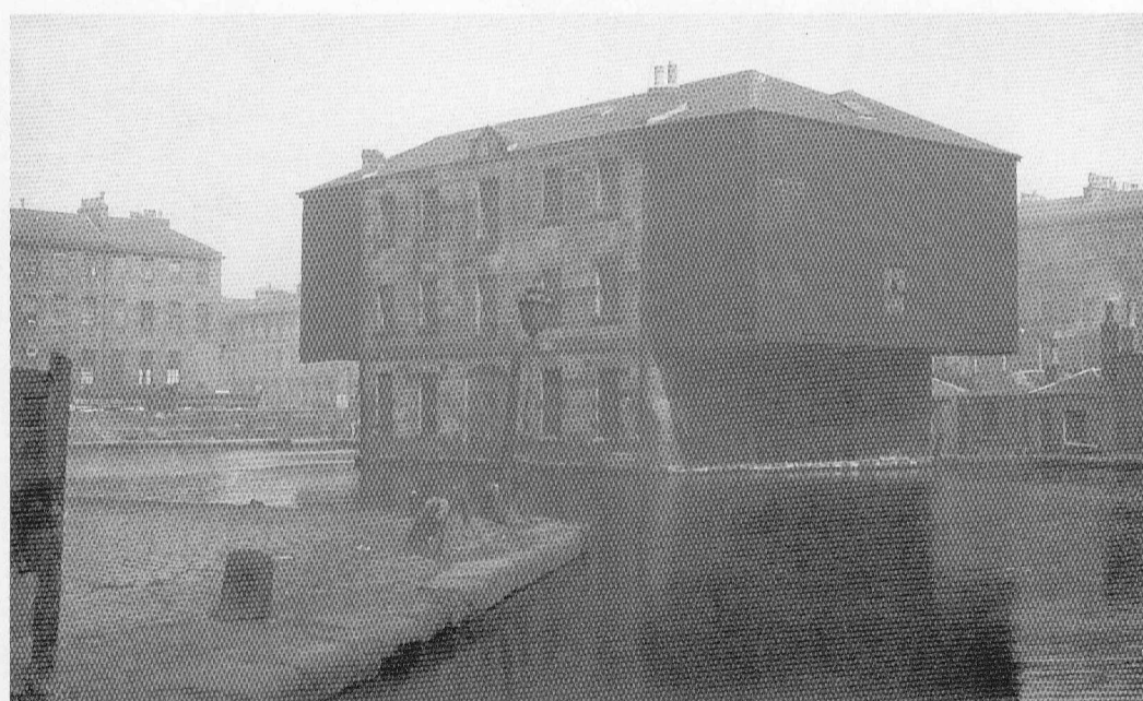
Edinburgh, Port Hopetoun, c. 1923; warehouse and quayside from south-west. (SC677924)
