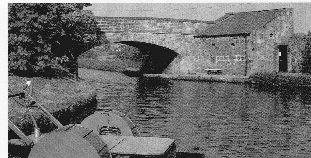
Powflats, Bridge No 23; bridge and associated building from south-east. (SC678606)
