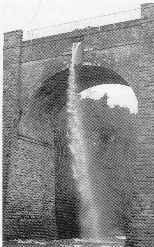
Almond Aqueduct; south face of arch over river with control sluice discharging surplus canal water. This overflow froze in February 1895, famously creating a 75-foot (23m) pillar of ice. (SC678656)
