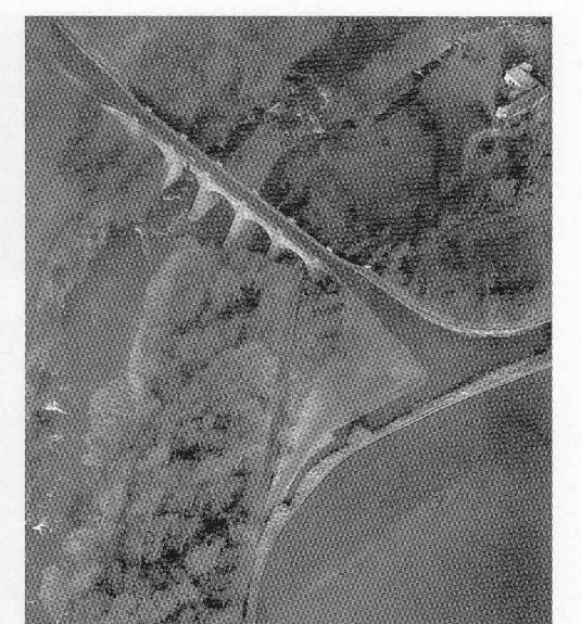
Almond Aqueduct: oblique aerial view showing feeder flowing into canal from bottom centre (south). (SC677934)
