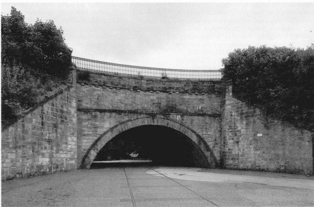
Kirkintilloch, Luggie Aqueduct; north face showing inserted level of later railway. (SC691359)
