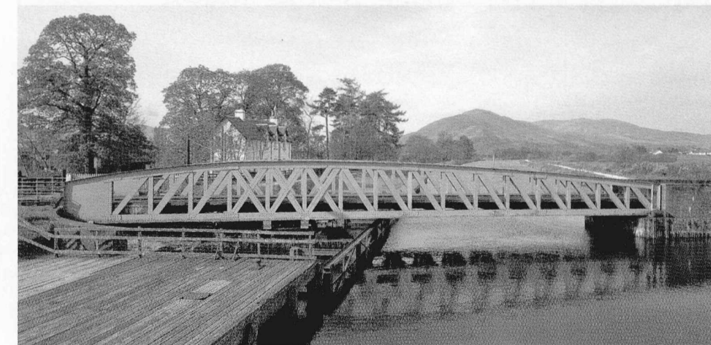
Banavie; steel bow-truss railway swing bridge over Caledonian Canal from north-east. (RCAHMS: D48394/CN)
