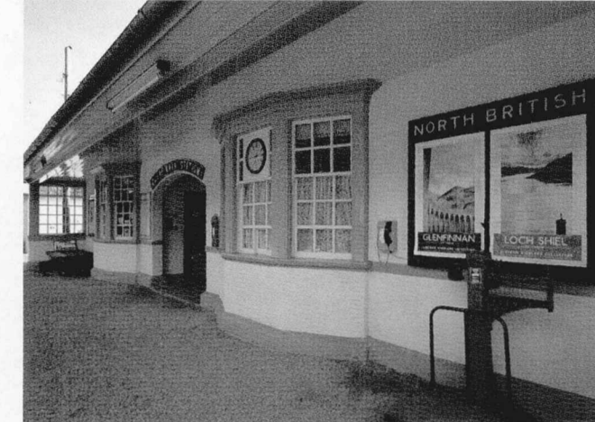
Glenfinnan Railway Station; former booking office, now a museum. (RCAHMS D48021/CN)
