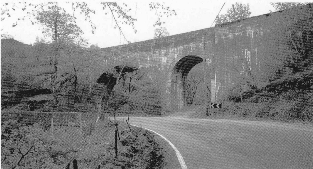
Larichmore Viaduct, from south. (RCAHMS: D48110)
