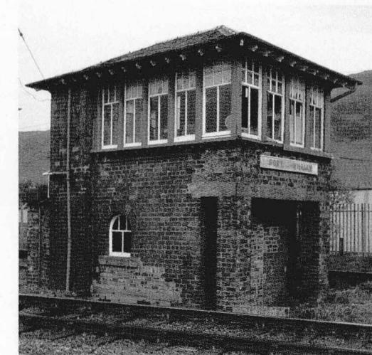
Fort William Junction; brick-built signal box from west. (RCAHMS: D48100/CN)
