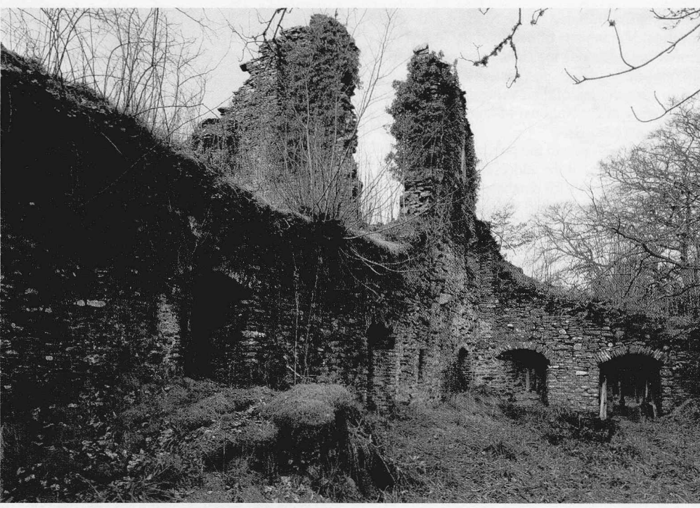
9 Corra Castle: view of the courtyard from the south. (SC877113)
