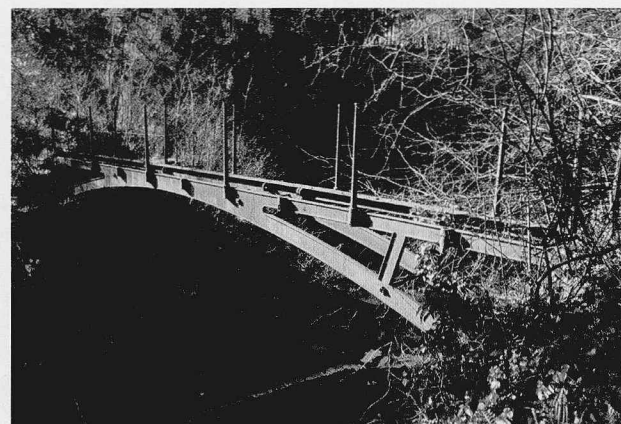
13 The cast-iron single-span bridge at Bonnington Linn was made by local engineering firm Paterson of Carmichael in the mid 19th century. (DP001869)
