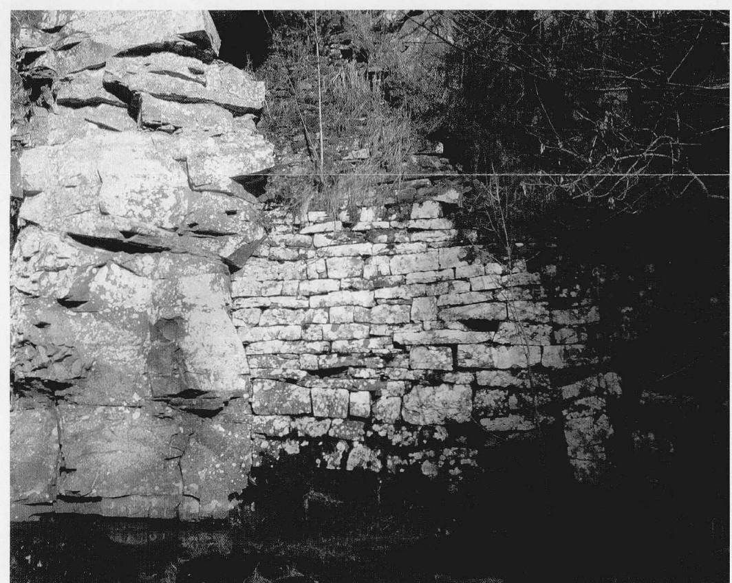
15 Lady Mary's Steps: construction detail. Now decayed and dangerous, these were built for Lady Mary Ross of Bonnington in 1829 to allow visitors access to the east bank of the river below Corra Linn. (SC877117)
