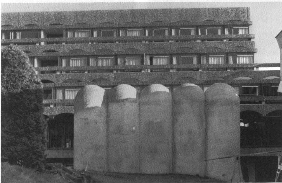
4.54. Main Block nearing completion, c.1966. Gillespie Kidd & Coia Archives
