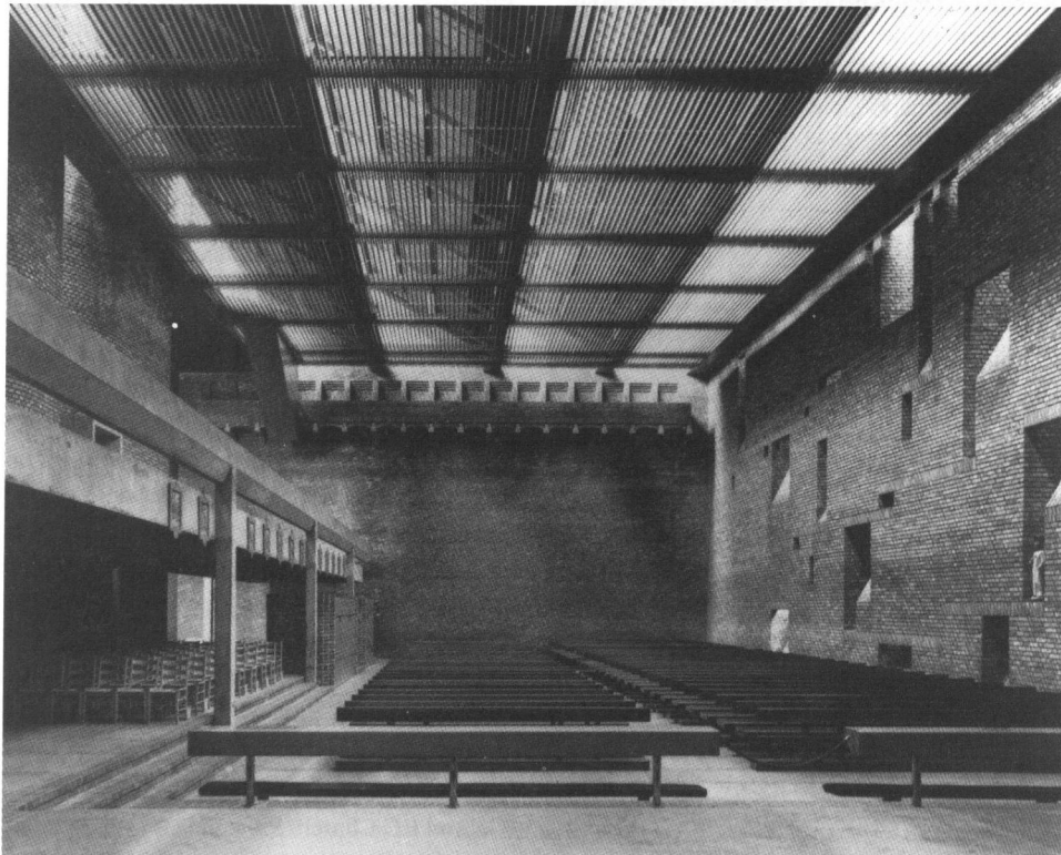
3.10. St Bride's, East Kilbride, by GKC, 1963-4. The firm's most important brick load-bearing church design. Diffused lighting from above, and through the carved openings in the thick brick walls, creates a spiritual and lofty interior. Sam Lambert
