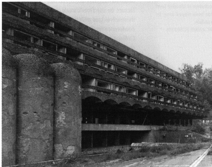
5.8. 1994 view of Main Block. RCAHMS [C50196]
