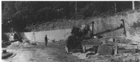
4.42 Construction of retaining wall in progress, April 1961. Scotus College [C67449]
