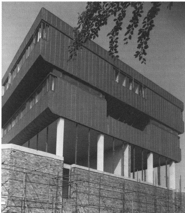
3.14 Our Lady's High School, Cumbernauld, by GKC, 1963-4. The sectional arrangement and layering of spaces is clearly visible in this view, taken during construction. Gillespie Kidd & Coia Archives
