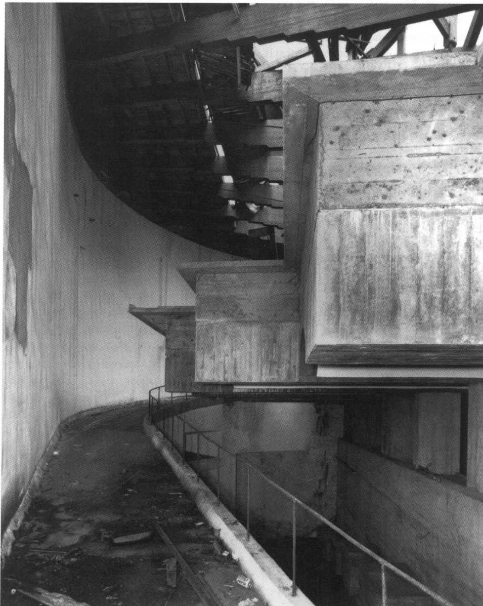
6.3. The sanctuary ramp, seen in ruins, 1994. RCAHMS [C50212]
