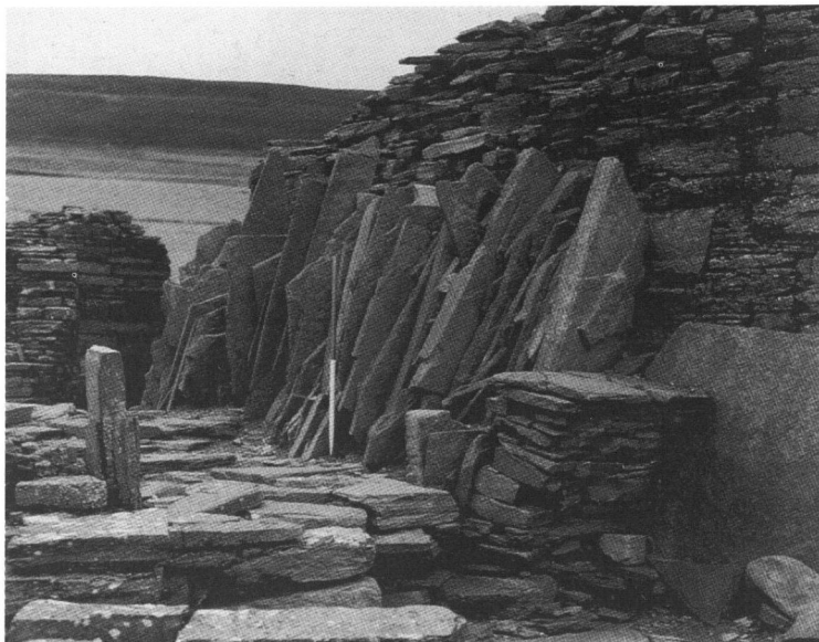
Buttressing was added outside the broch to prevent collapse
