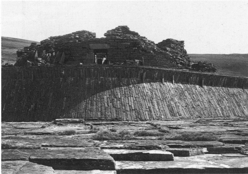
A modern sea-wall protects the broch of Midhowe from coastal erosion
