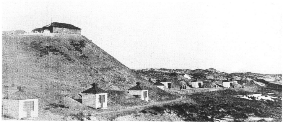
Plate 23: View of original Dynamite cartridging huts situated beneath nitroglycerine hill (left), illustrating the wooden construction and layout of the buildings, circa 1880, (ICI Explosives, C62976)
