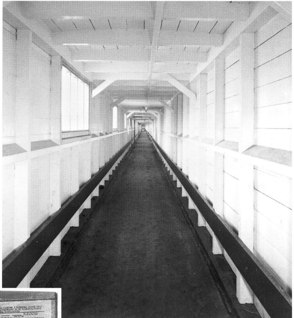
Plate 53: Interior view along covered walkway No.4 within the Detonator Department, showing a long section of wooden walkway typical of several areas of the factory, 1995. One of the main purposes of these enclosed corridors was to prevent sand from blowing or being carried into production areas. (RCAHMS, C38948)
