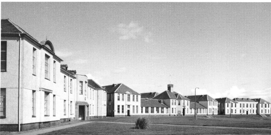
Plate 48: View from north west of central range of Offices, Laboratories and Library, incorporating what is now referred to as Nobel House. These buildings date from the formation of ICI in 1926, and were built to house ICI's research centre, comprising the Research Department Headquarters, and including an office for the Research Manager, and associated administrative offices, laboratories, and the library. 1995 (RCAHMS, C38963).
