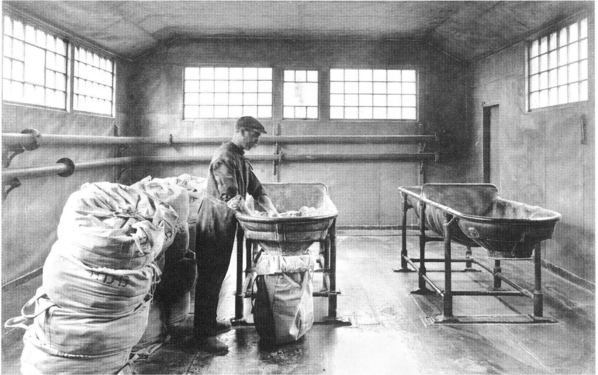
Plate 35: (above) Interior view in Propulsives Department, showing Cordite paste mixing house, circa 1925 (ICI Explosives, C65546)
