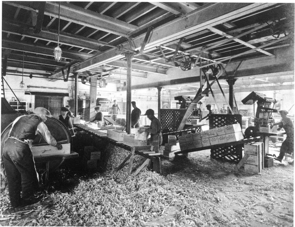
Plate 24: (below) Interior view of Box Factory, showing nailing and trimming machines, circa 1925 (ICI Explosives, C65560)
