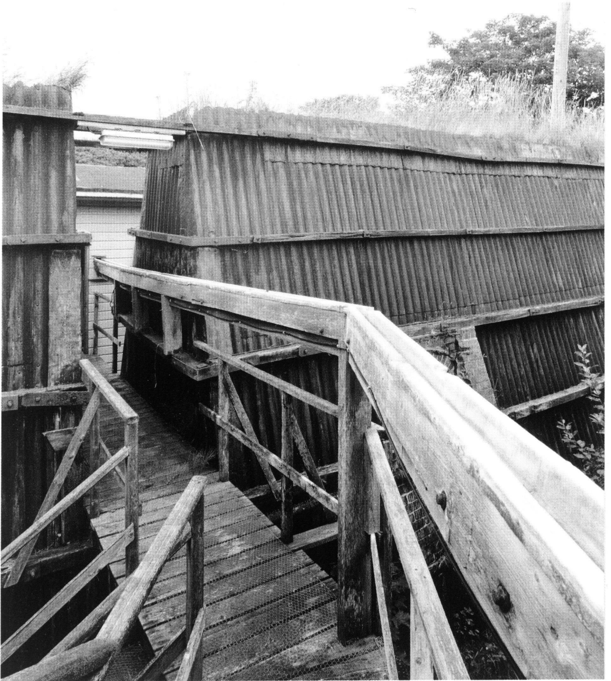
Plate 57: View of AC2, a 'C' House on Nitroglycerine Hill No.2, showing the wooden gangway and lead-lined gutter approaching through a gap in the Chilworth Mound, which isolates the building, 1995 (RCAHMS, C60084)
