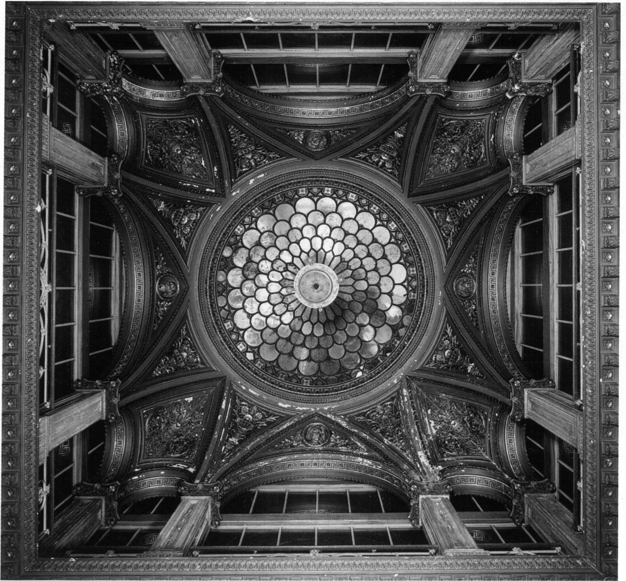
22 Park Circus, Glasgow: cast-iron cupola, the crowning glory of a rich mid-Victorian interior
