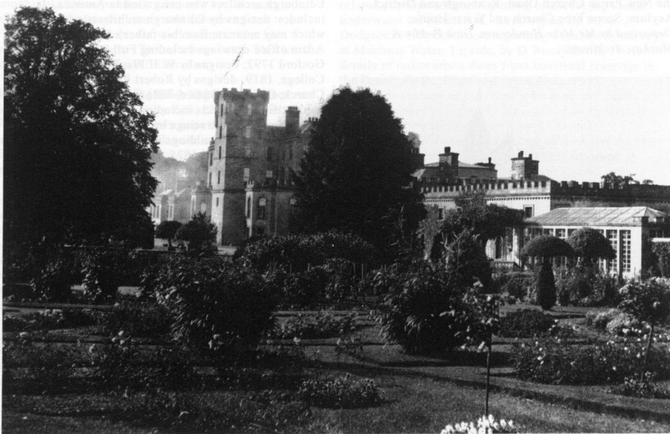
View of Gordon Castle, Moray, c.1910, from Rossie Priory album. Castle now mostly demolished. [C 47414]
