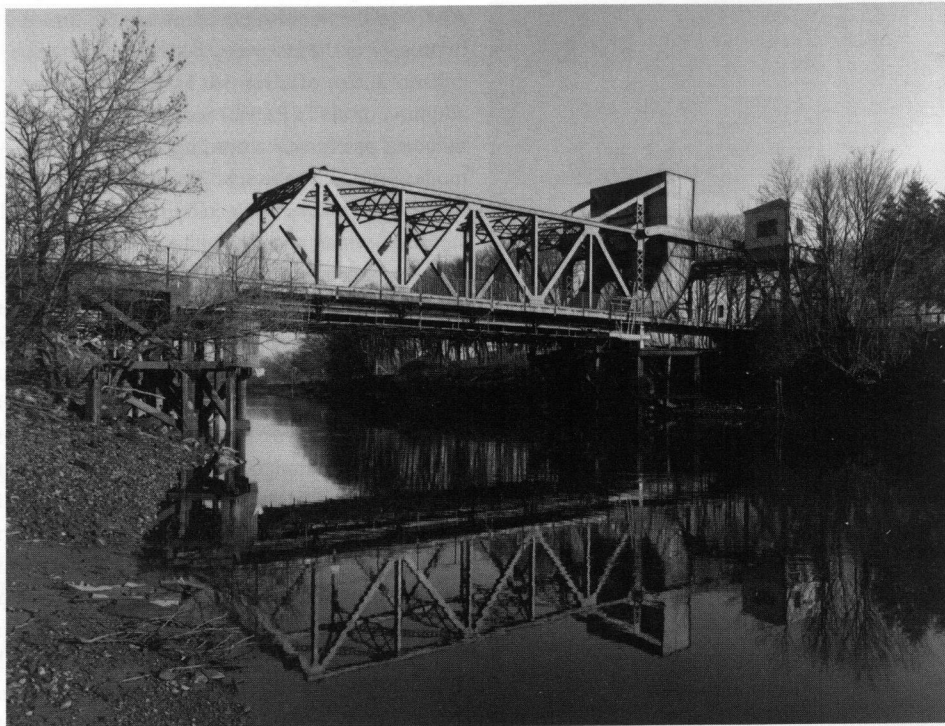
Rolling Lift Bridge (over White Cart), Inchinnan, Renfrewshire. [D 06576]
