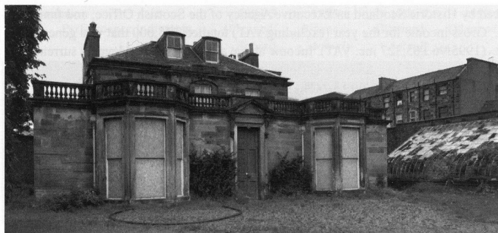
Fairfield House, Dalkeith, Midlothian; view showing the original house, the mid nineteenth-century extension, the hot house and the earlier garden wall. [C 69375]
