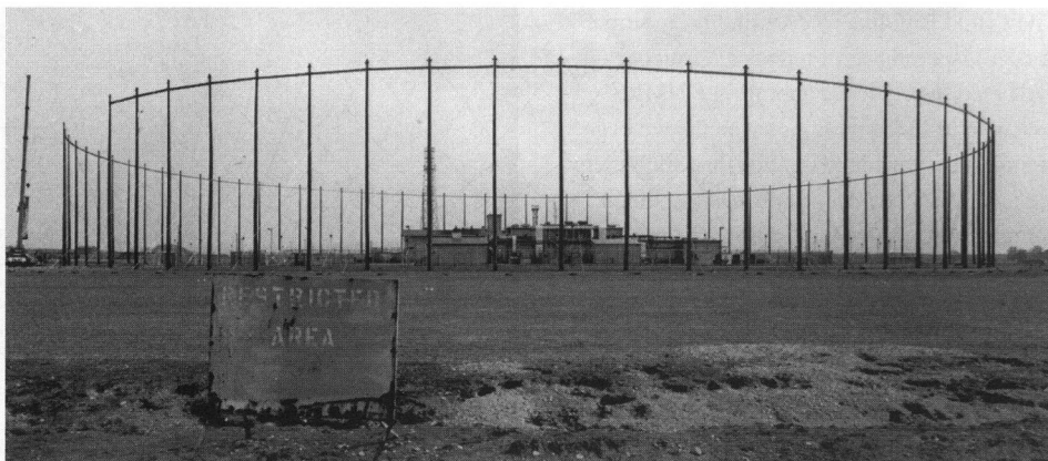
Communications Intercept Station, Edzell Airfield. The Wullenwrecker Array (now demolished), known locally as the 'elephant's cage', was used to detect weak signals from clearly defined directions. [D10669]
