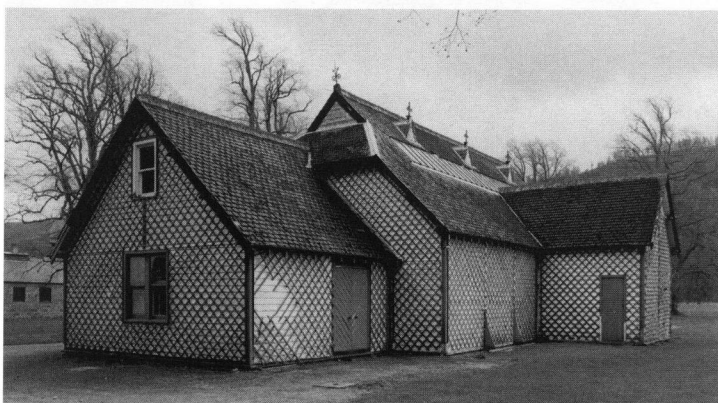
Mar Lodge, Ballroom: exterior and interior views. [D12135, D12145]
