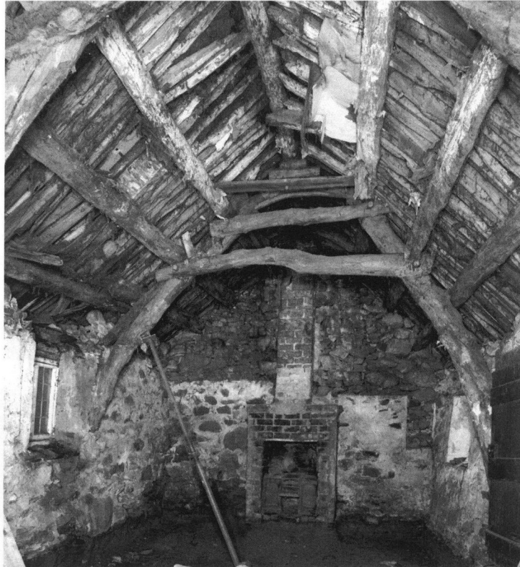
Briar Cottage, Lochearnhead: interior view showing cruck-framed roof structure. [D25535]
