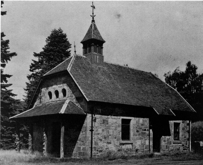
14 Exterior from S
